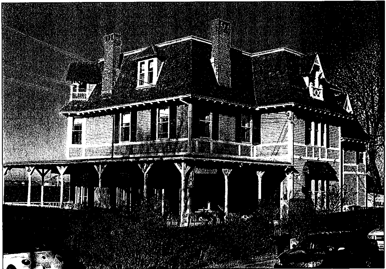
Sanford-Covell House (1869/1870), 72 Washington Street. Photograph by Jeffrey D. Emidy, December 2006.
