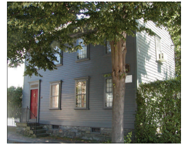
Wooden clapboards are the most common exterior treatment on Colonial-Era homes in Newport. With proper care and maintenance, wooden clapboards can last for generations.
