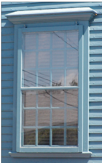
Well-chosen storm windows have minimal visual impact on the original primary windows they are protecting. This example, found on one of Newport's Colonial-Era homes, is a perfect example of a well-fitted and visually harmonious storm window.
