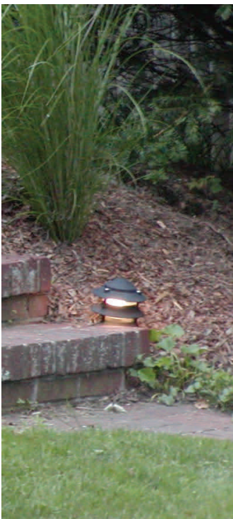
Foot height lighting is a very discreet way to illuminate pathways and steps, increasing safety with minimal visual compromise to the site.
