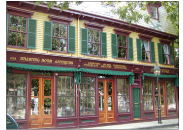
A unifying façade rhythm is created by the pattern of entries, display windows and retractable awnings of this sensitively rehabilitated commercial building.
