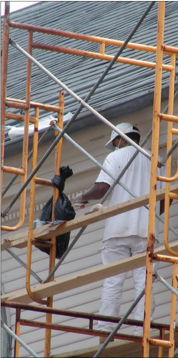
Great care should be taken when removing old paint, especially if you suspect that there is lead in it. This man, working high above the ground on Trinity Church, is taking proper precautions while removing old paint by wearing a face mask and gloves. Using a hand-scraping technique is the best way to remove paint to minimize the chance of damaging historic
