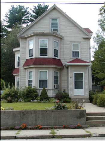
This photo shows a case where both vinyl siding and inappropriate replacement windows have compromised the integrity of a building's historic character.
