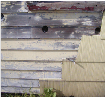
Modern siding stripped away to reveal older wooden clapboards. Depending on their condition, the newly-uncovered clapboards might be sound enough to be refinished and repainted, restoring this home to how it looked at one time in the past.
