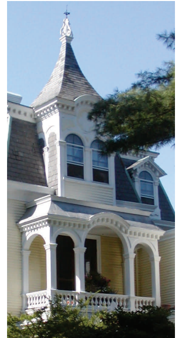
A finely-detailed and well-preserved second story balcony overlooking Kay Street.
