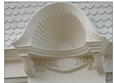
Wooden features such as this exquisitely detailed carved shell motif should be carefully maintained and preserved. Such skilled craftsmanship like this is very rare today.
