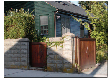
A low wall constructed of granite with wooden gates provides privacy
