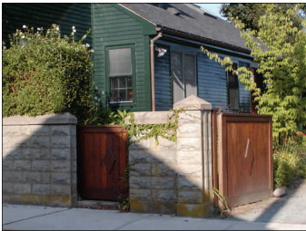
A variety of fences and walls in a variety of materials are found throughout the district. Decorative gates embellish some.
