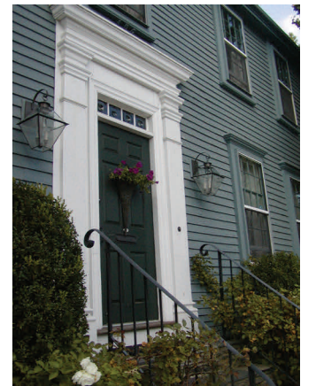
Distinctive features, such as the transom lights above this colonial doorway, should be kept intact whenever possible. Many colonial-era homes in Newport feature elaborately carved ornamental crowns and door surrounds.
