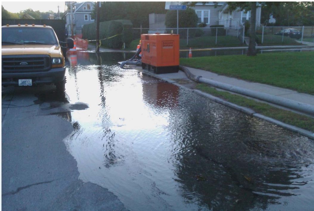
Intersection of Wellington Avenue and Marchant Street during a High Tide on 10/07/2011
