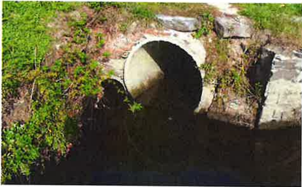
Figure 2. Drainage Outfall Locations at the Moat
