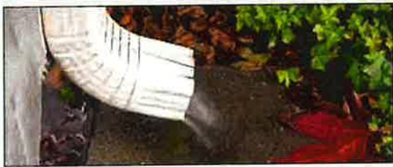
Reroute your downspout so your yard or rain garden absorbs and filters the runoff from your roof.
