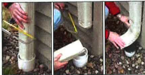
Disconnecting your downspout is a simple and effective way of reducing stormwater runoff. (Photo from grandbuilding.ca )
