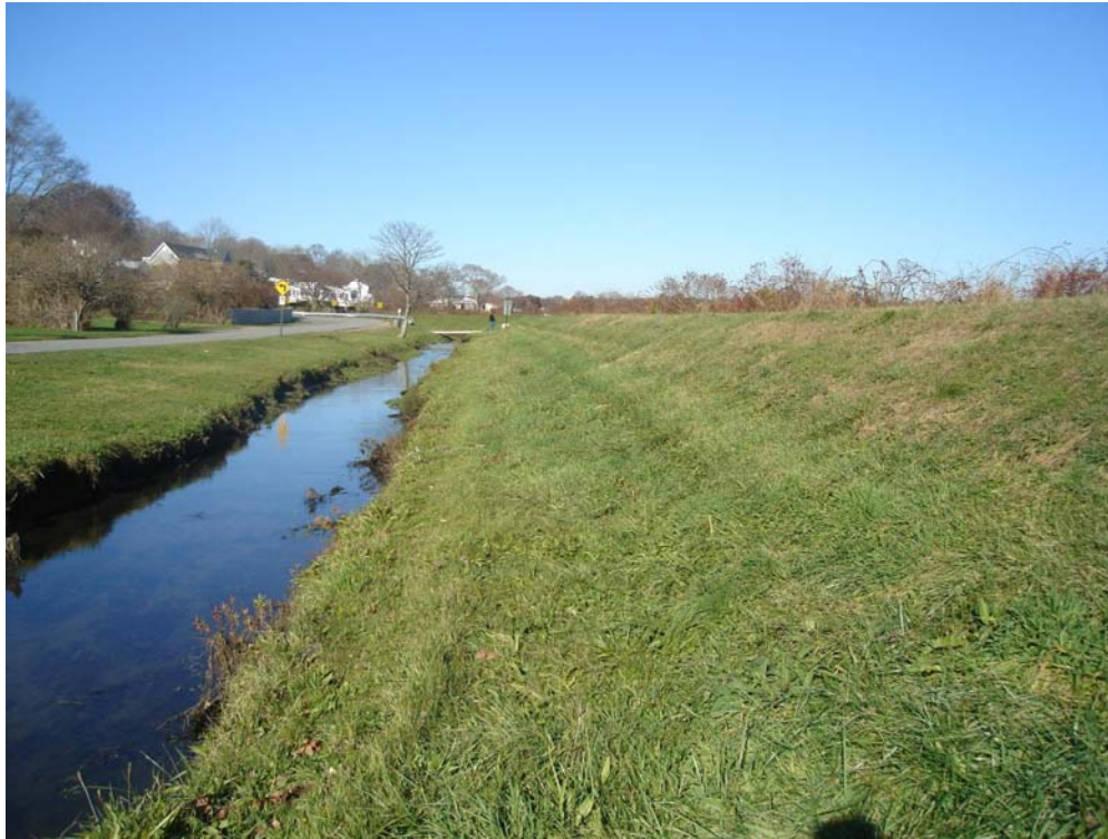
Sta. 36+36: Photo of Moat along Old Beach Road (Looking in Upstream Direction)
