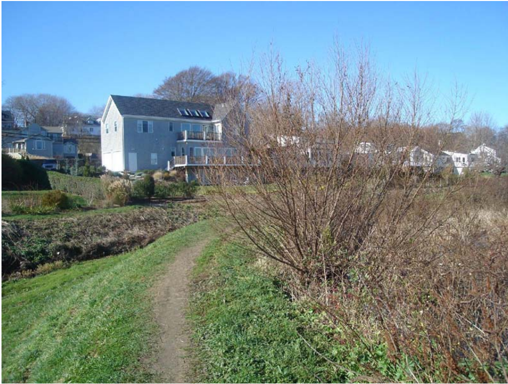
West Embankment – Footpath on embankment crest
