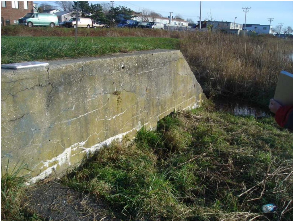
North Pond Primary Spillway - Cracking and efflorescence on face of left abutment
