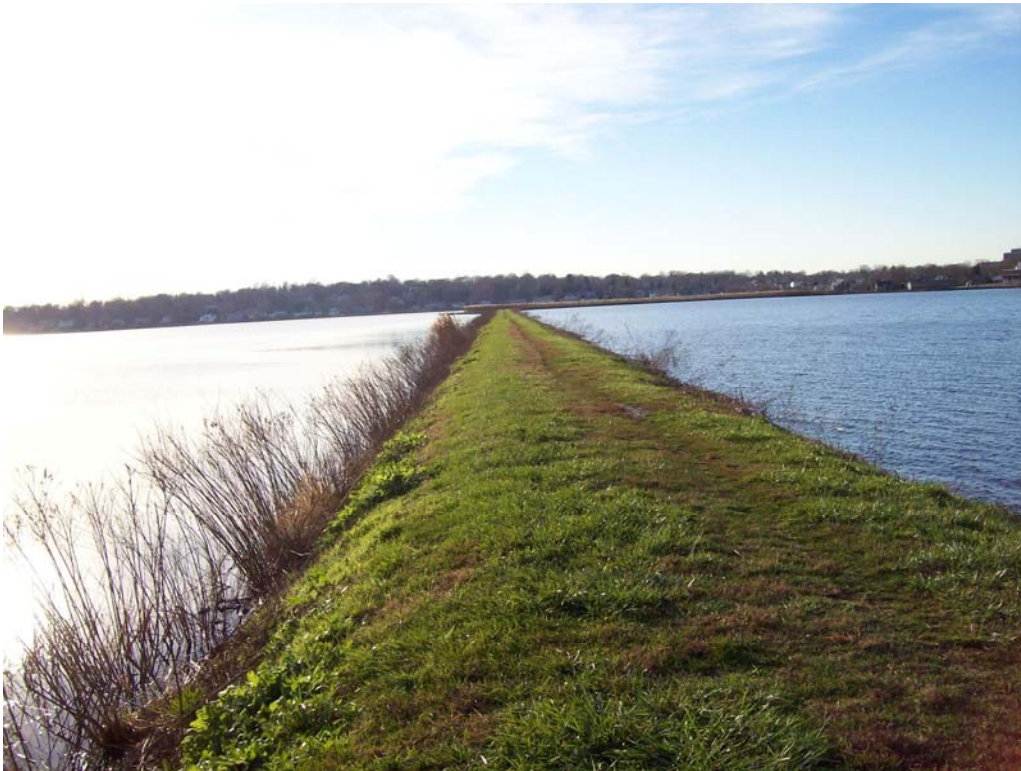
South Pond/North Pond Dividing Embankment – Footpath on embankment crest
