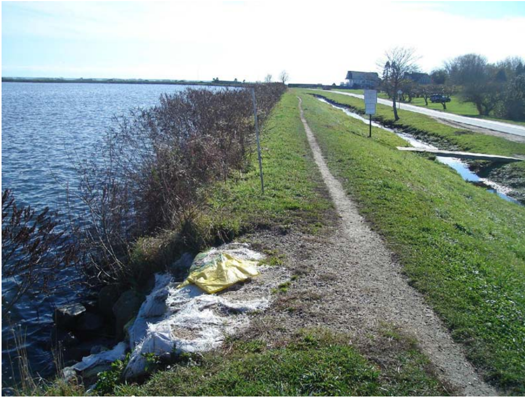
West Embankment - Repair area on upstream slope
