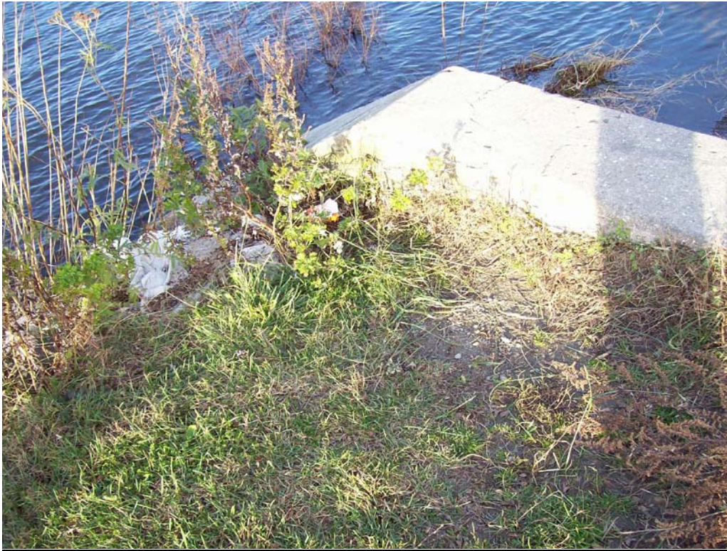
North Pond Primary Spillway – Runoff channel adjacent to upstream right abutment
