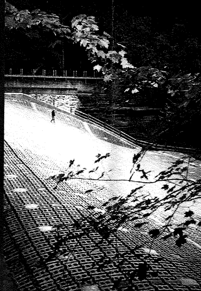
ARTICULATING CONCRETE BLOCK REVETMENT SYSTEM
