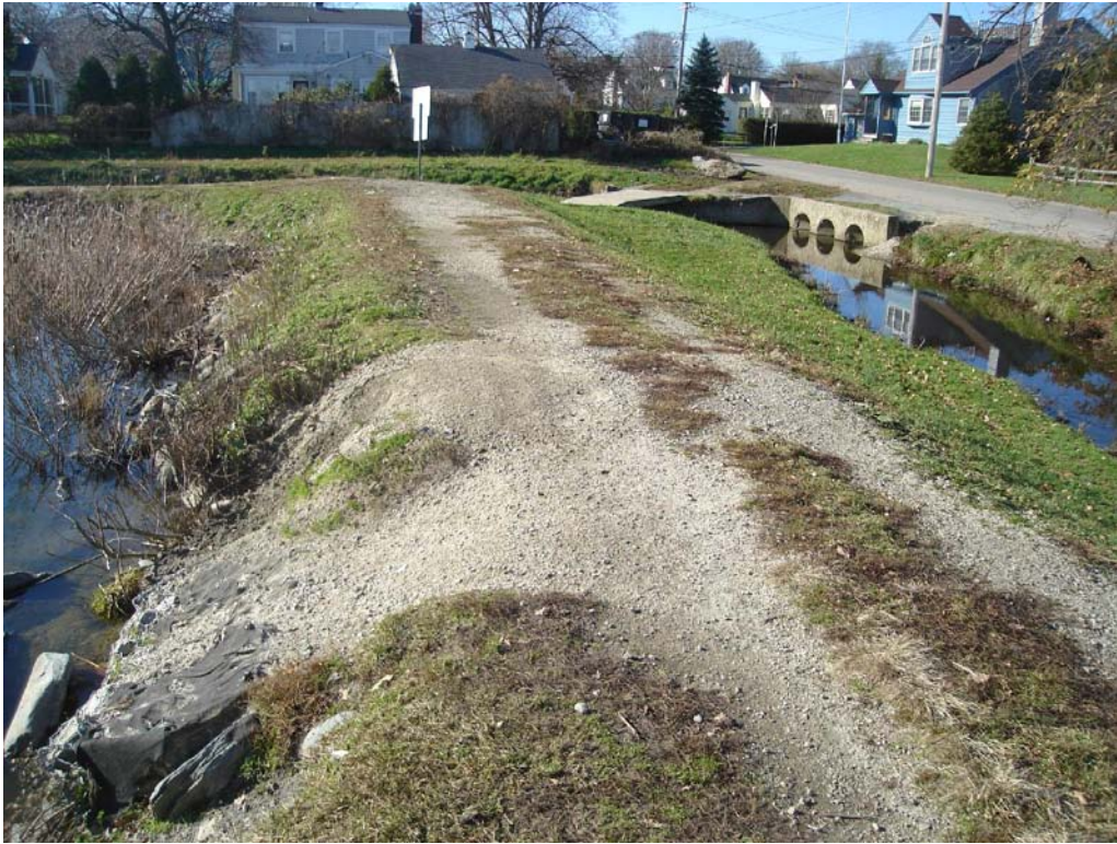
North Embankment – Scarp repair on upstream slope
