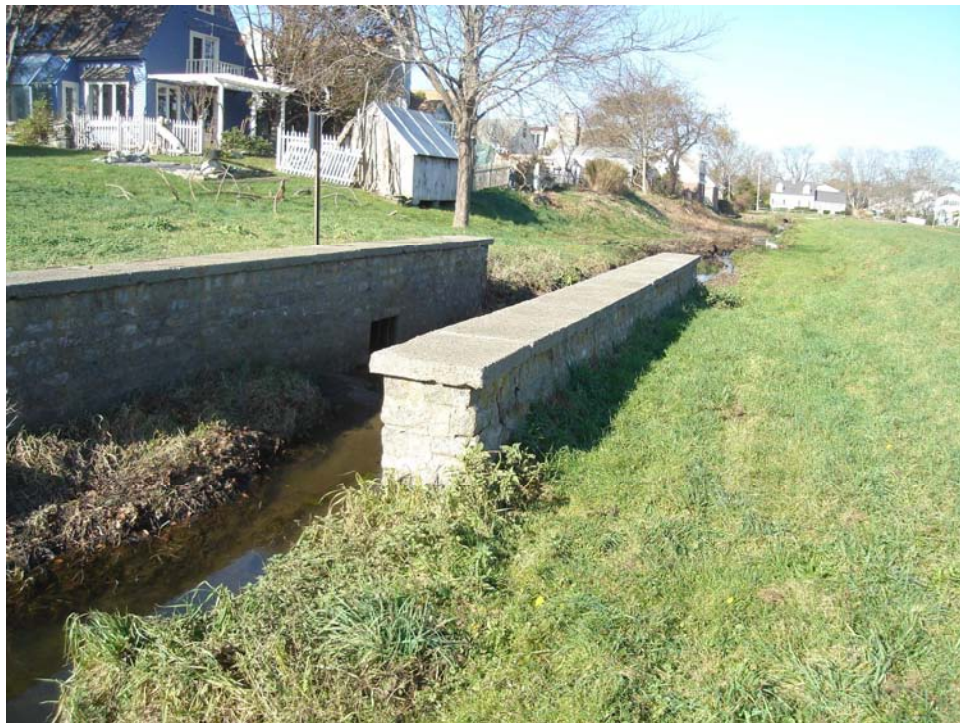
Sta. 57+19: Photo of Moat and Overbank Areas (Looking in Upstream Direction)
