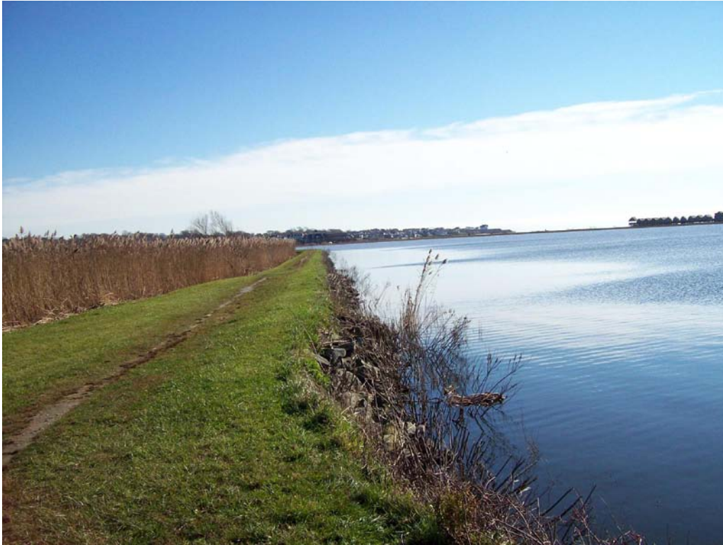
North Embankment – Riprap protection on upstream slope
