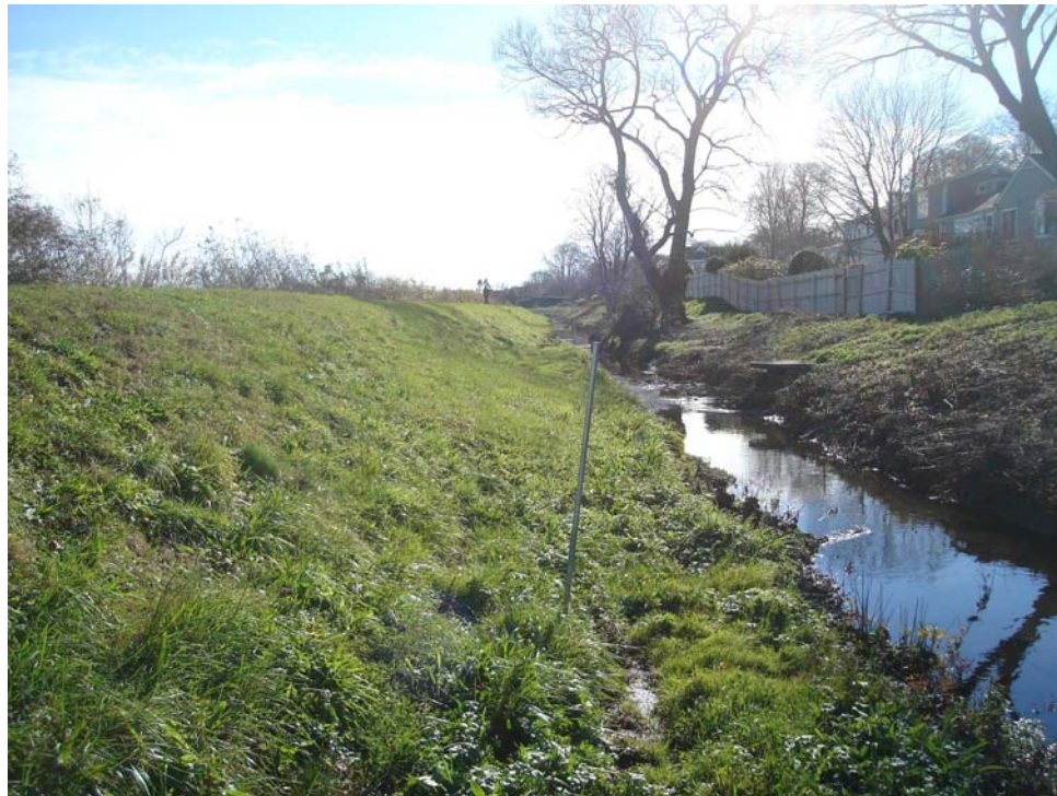
Sta. 50+21: Photo of Moat and Overbank Areas (Looking in Downstream Direction)
