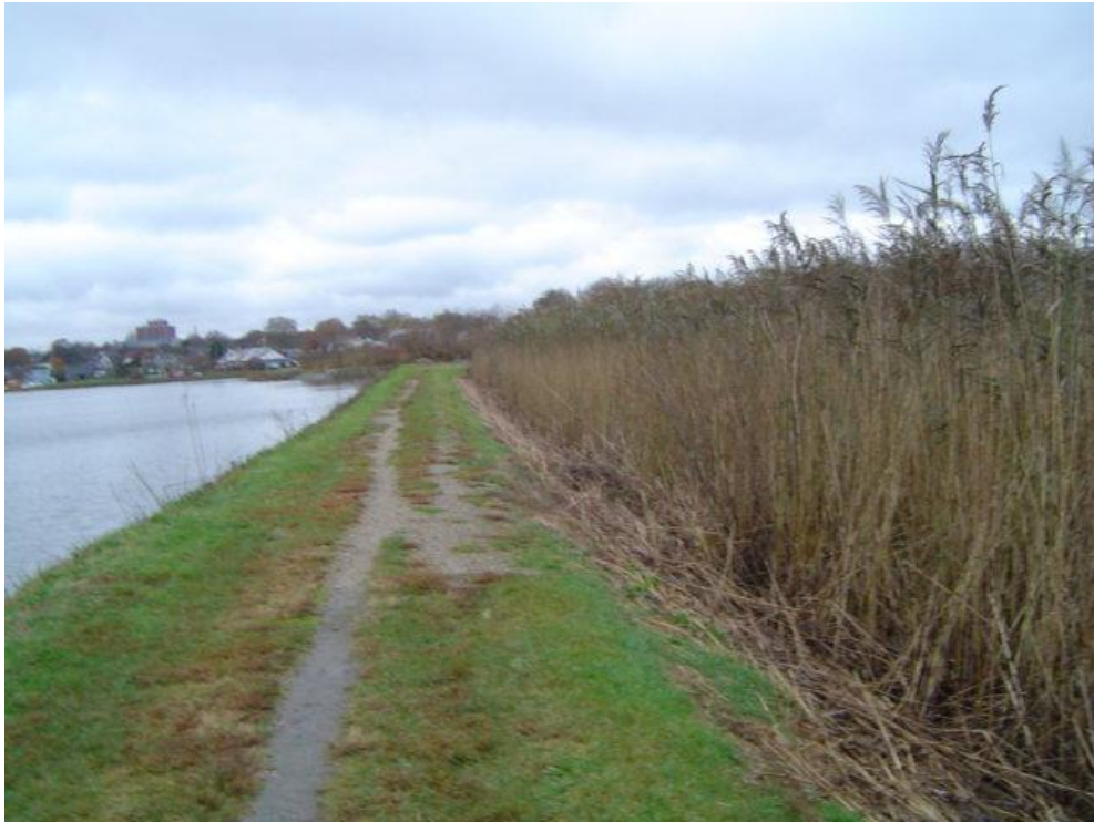
Sta. 84+15: Photo of Pond Embankment and Low-Lying, Marsh Area Storage (View of Left Overbank Area Looking in Downstream Direction)
