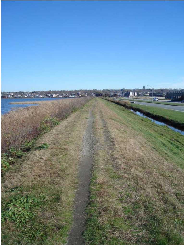
South Embankment - Footpath on embankment crest
