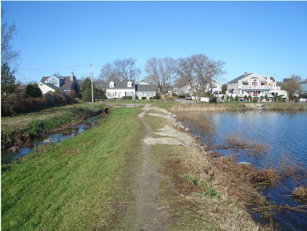
West Embankment – Repaired scarps on upstream slope
