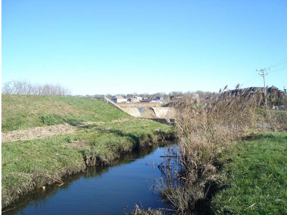
Sta. 5+55: Photo of Moat along Memorial Boulevard at Confluence with Spillway Channel from South Easton Pond (Looking in Downstream Direction)
