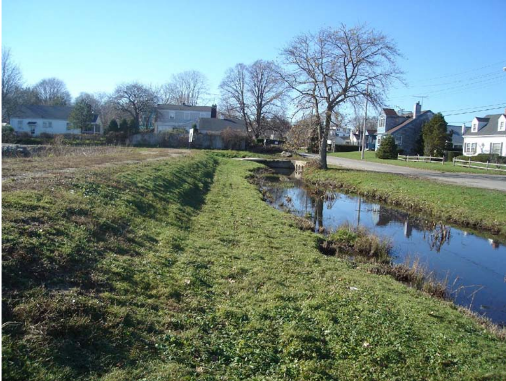
Sta. 65+34: Photo of Moat and Left Overbank Area along Ellery Road (Looking in Downstream Direction)
