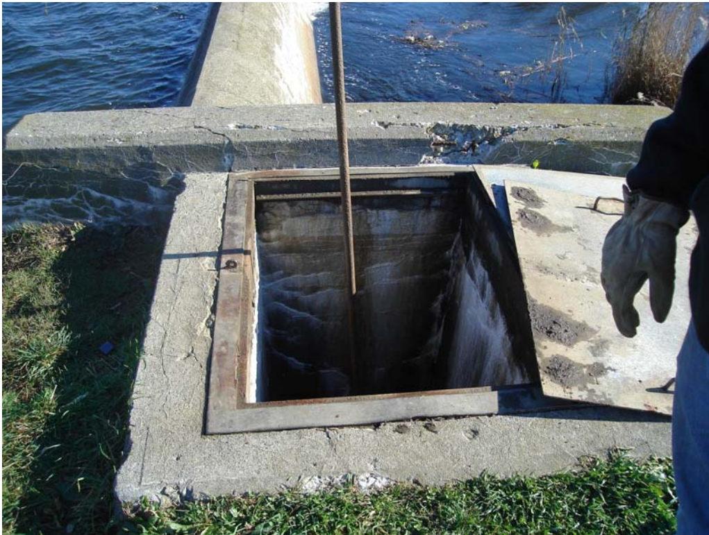
South Pond Spillway - drawdown structure chamber
