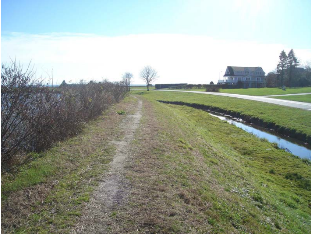
West Embankment - Footpath on embankment crest
