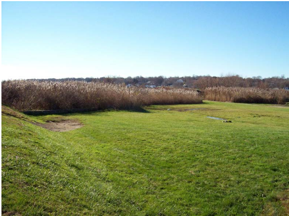
Sta. 77+82: Photo of Moat Right Overbank Area (Adjacent to Water Treatment Facility)
