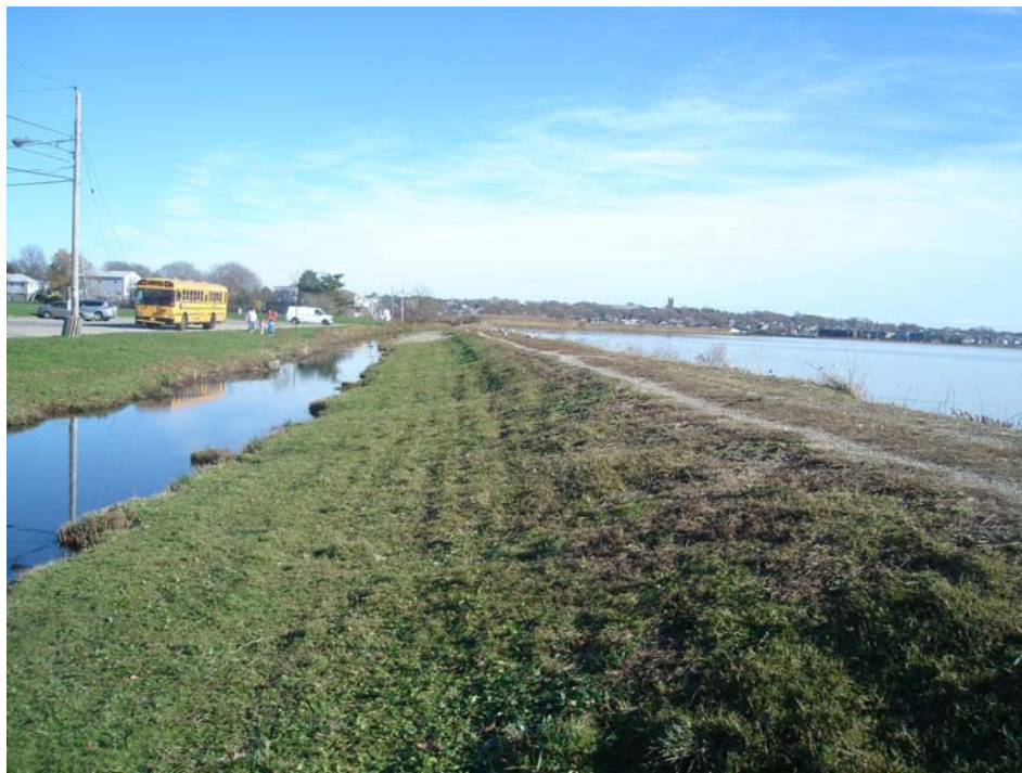
Sta. 65+34: Photo of Moat and Left Overbank Area along Ellery Road (Looking in Upstream Direction)
