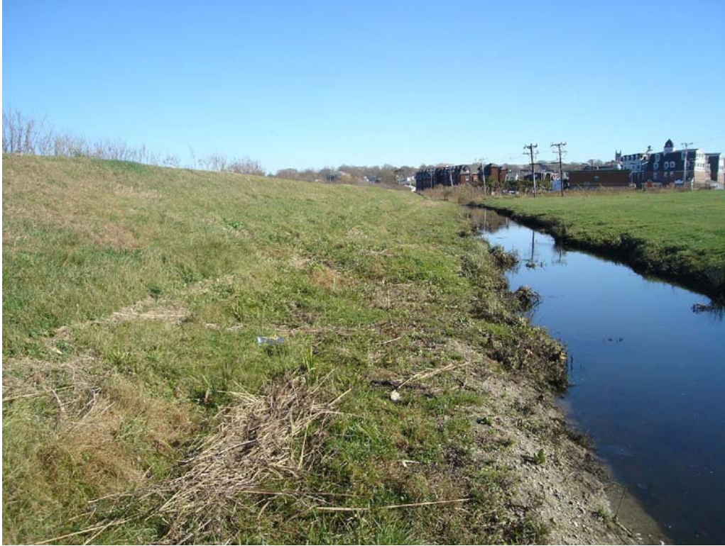
South Embankment – Narrow bench along downstream toe of slope
