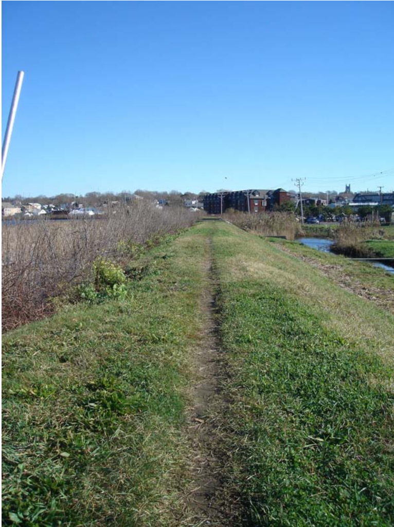
South Embankment - Footpath on embankment crest
