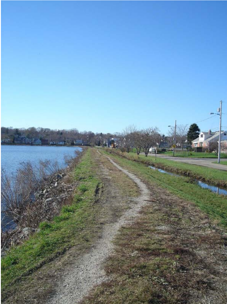
North Embankment – Footpath on embankment crest
