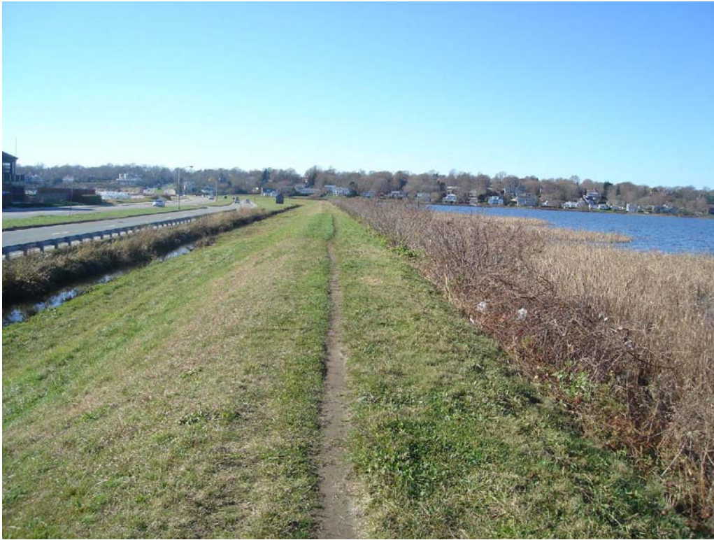
South Embankment - Footpath on embankment crest
