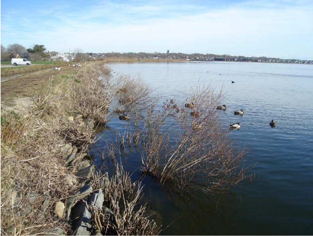
North Embankment - Riprap protection on upstream slope
