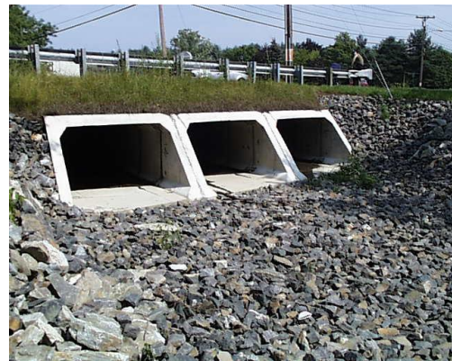
Photograph 20: Sample Photograph of Box Culverts
