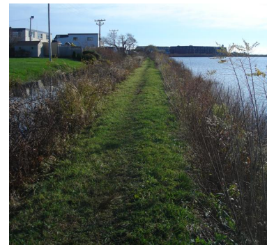
Photograph 1: Vegetation on East Embankment
