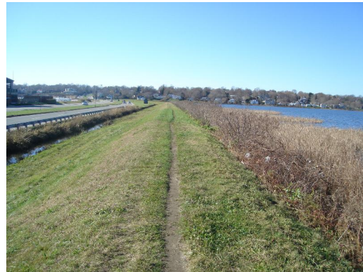
Photograph 14: Worn Footpath on Crest of South Embankment
