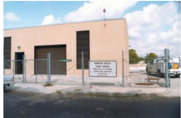
Photograph 21: Sample Photograph of Pump Station
