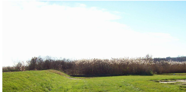
Photograph 2: Vegetation in North Pond Emergency Spillway Channel
