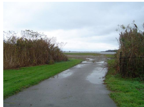
Photograph 18: Paved Access Path at Sta. 77+65
