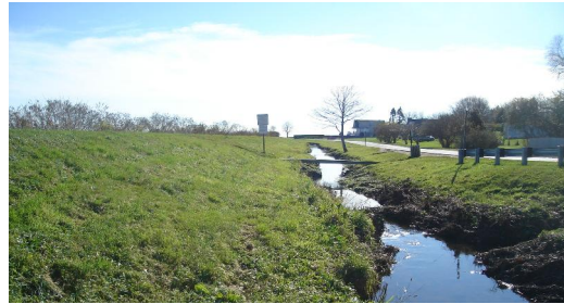
Photograph 10: Moat Scouring and Encroaching along West Embankment
