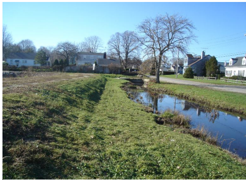
Photograph 15: Moat Along Ellery Road
