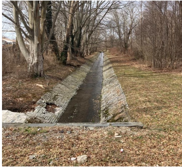
Figure 2-5. City-Owned and Maintained Malbone Channel ( photo taken in February 2022 )
