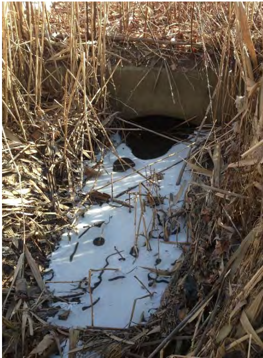
Photos 8-9: State drainage channel west of State 138/238 looking east at downstream headwall of twin 60" pipe culverts, vegetation and sediment visible (01/09/2014)
