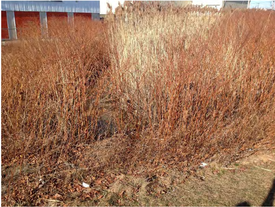
Photo 7: State drainage channel west of State 138/238 looking northwest from headwall of twin 60" pipe culverts (01/09/2014)
