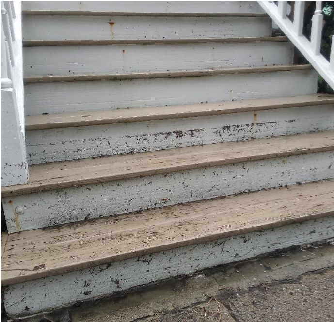
Photo 16: Resident provided photo of high-water mark due to an event on 9/13/2022, taken at 32 Halsey St
