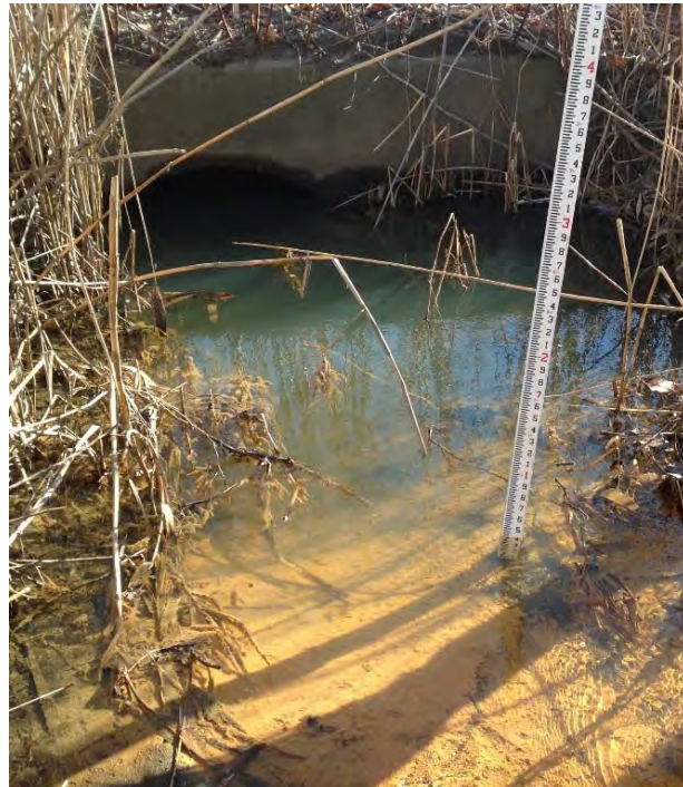
Photos 8-9: State drainage channel west of State 138/238 looking east at downstream headwall of twin 60" pipe culverts, vegetation and sediment visible (01/09/2014)
