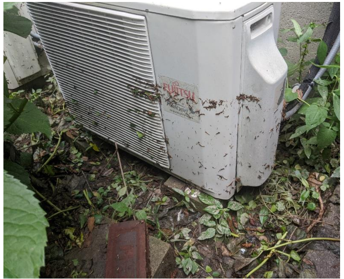
Photo 14: Resident provided photo of high-water mark due to Tropical Storm Ida (9/1/2021 – 9/2/2021), taken at 50 Halsey St
