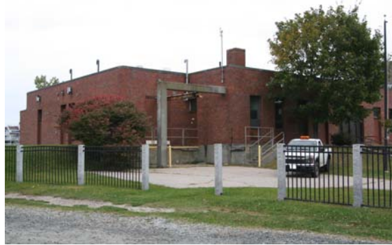
Wellington Ave. CSO Facility
