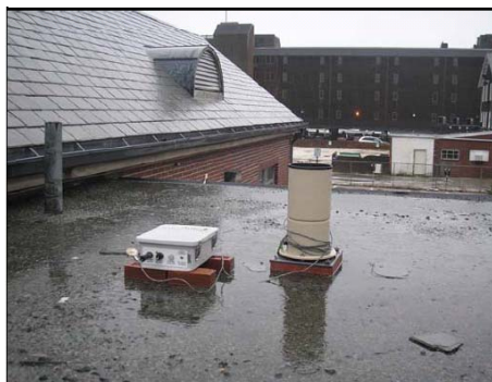
Rain gage at Long Wharf Pump Station
