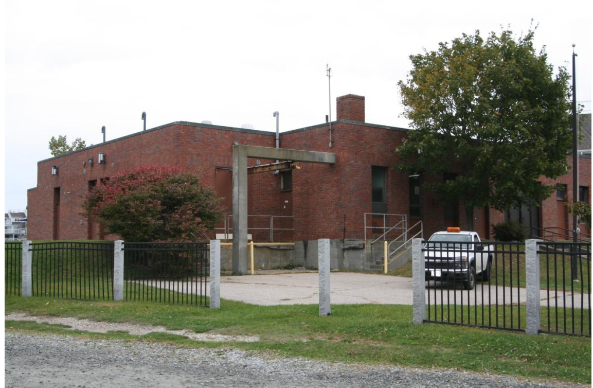
Wellington Ave. CSO Facility
