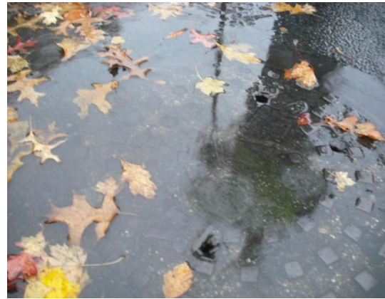
Vented manhole cover
