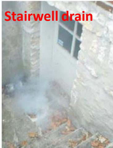
Service lateral defects
