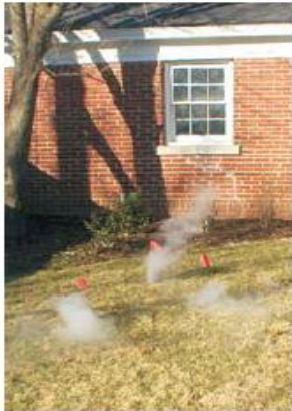
Service lateral defects
