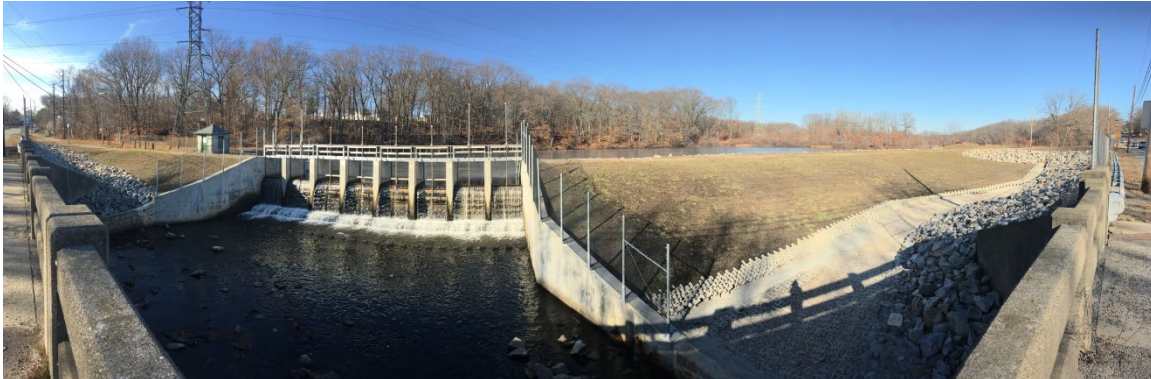
Figure 27 – Example Spillway Configuration for Adaptive Spillway Capacity
