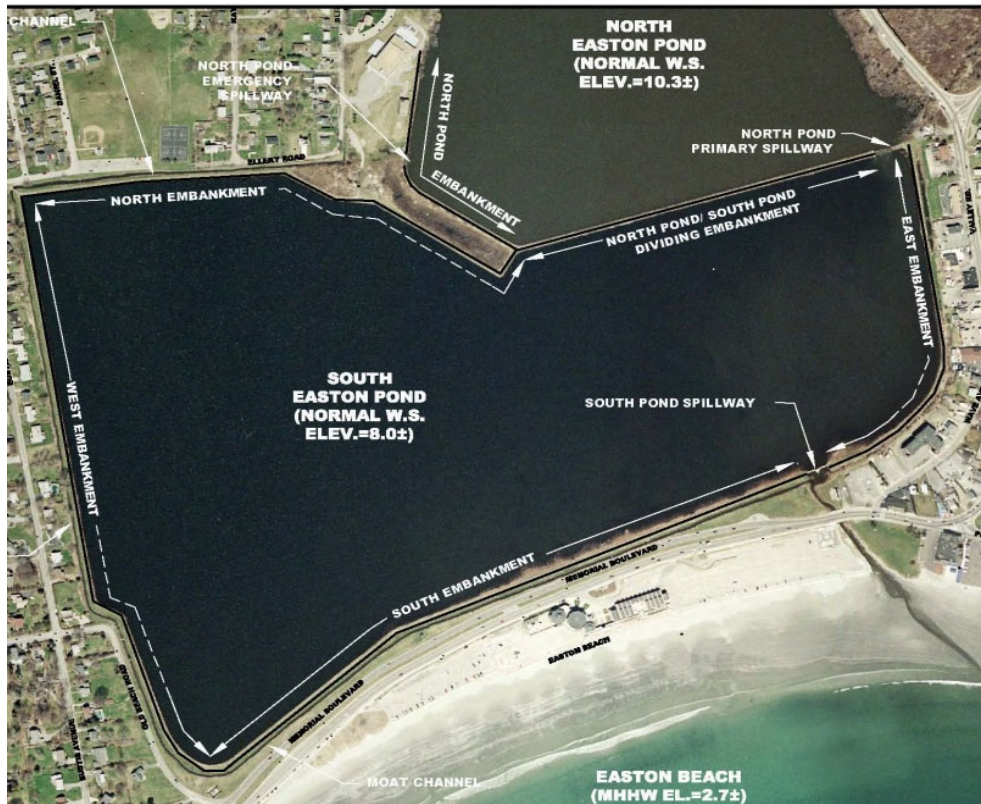
Figure 6 – South Easton Pond Dam Overview
