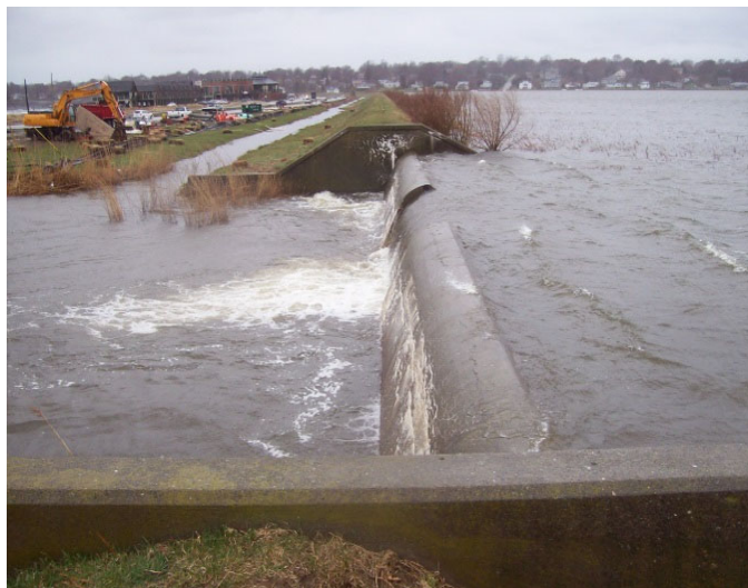
Figure 4 – South Easton Pond Dam Spillway Structure
