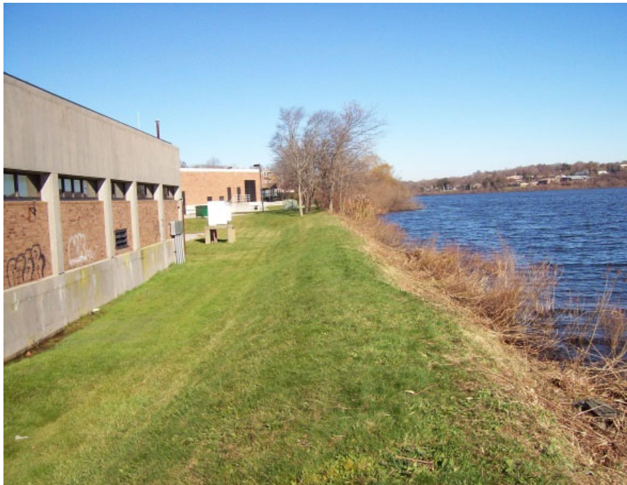
Figure 5 – North Eastern Pond Dam West Embankment
