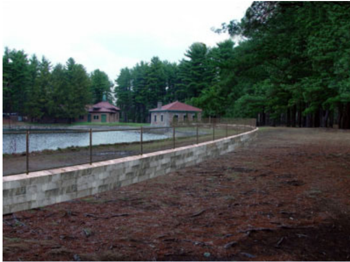
Figure 29 – Parapet Wall on a Dam http://www.mwra.state.ma.us
