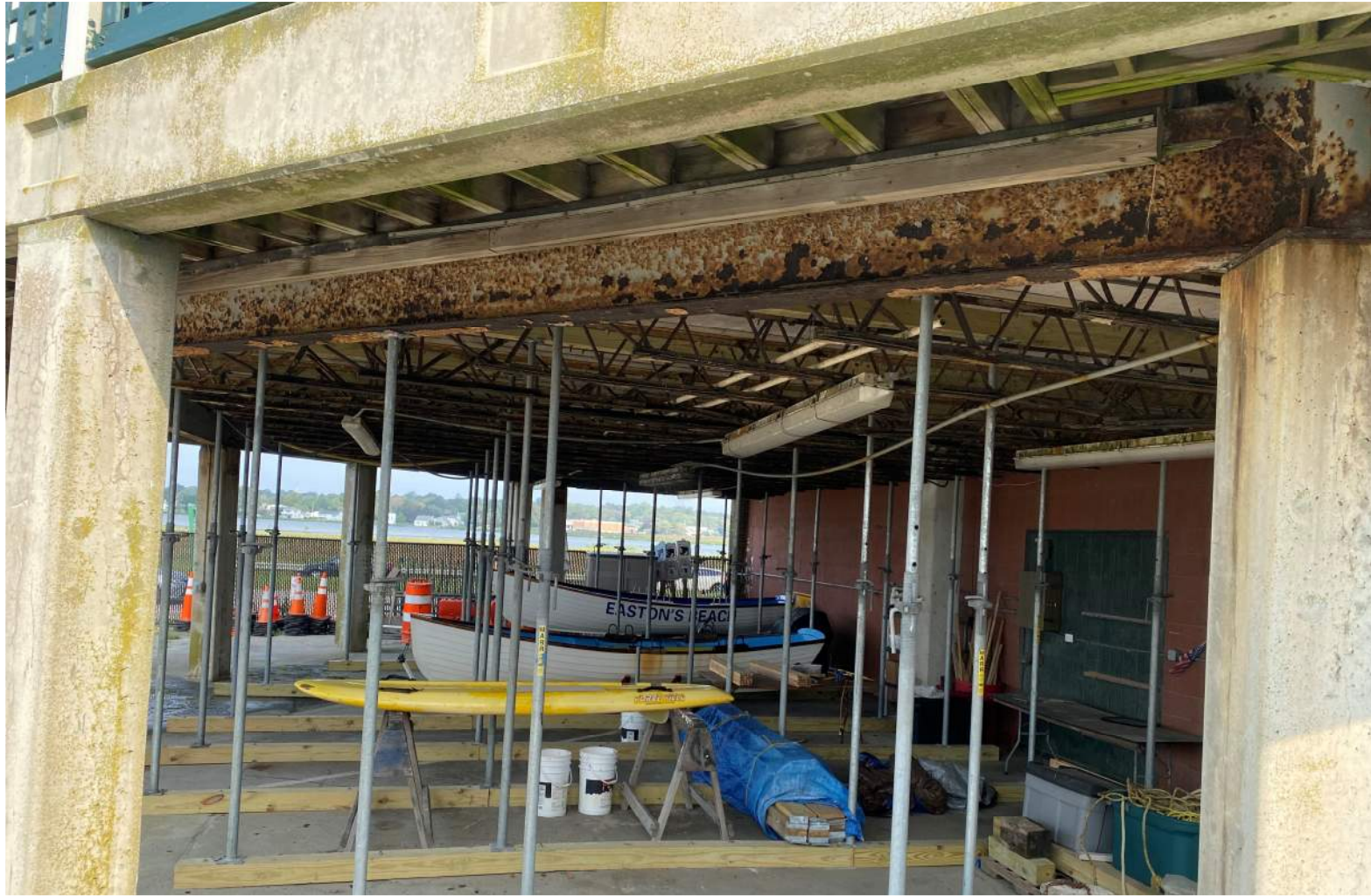
CAROUSEL BUILDING – TEMPORARY STRUCTURAL REPAIRS
