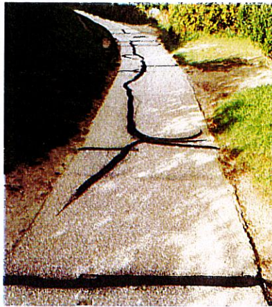
Figure 11: Crack Filling on Walk
