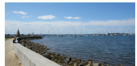
King Park Seawall
