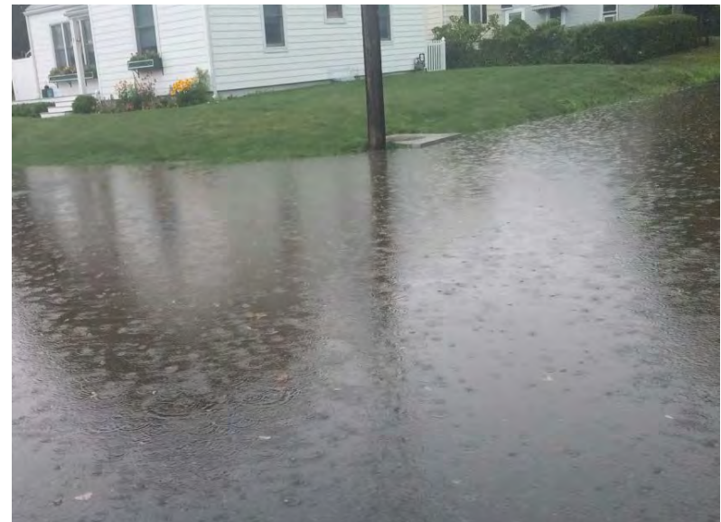
Flooding on Whitwell Avenue, August 15, 2012 6
