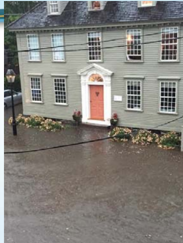
July 1, 2015 – Bridge Street between America's Cup and Thames Street ~ 1 ¼" rainfall in 1 Hour coinciding with High Tide
