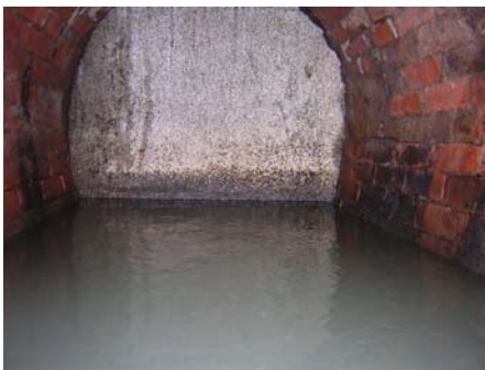
PHOTOGRAPH 3.1: Upstream view of 42-inch Restrictor Plate at Wellington Avenue Diversion Structure
