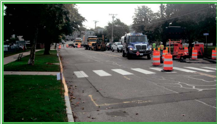
Wellington Avenue Construction
