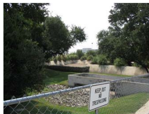
Structural Sand Filter
