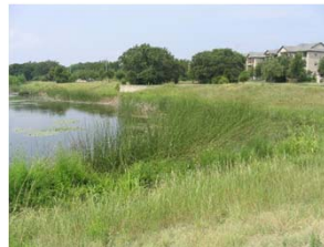
Suburban Detention Basin
