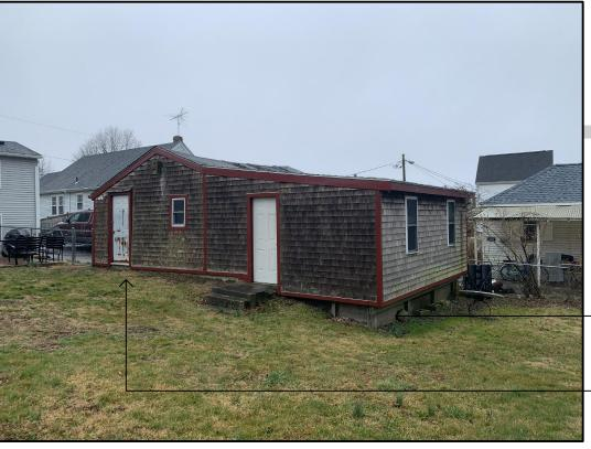
EXISTING STRUCTURE BUILT ON 4X4 POSTS.
