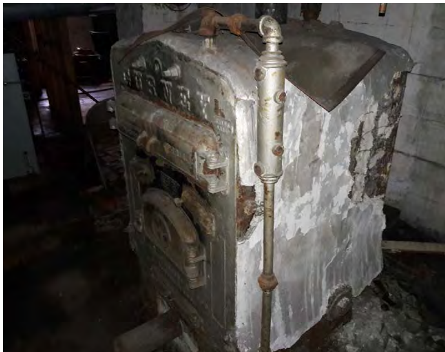
View of the furnace located in the basement of Building #1 wrapped in a potential asbestos containing material (ACM).
