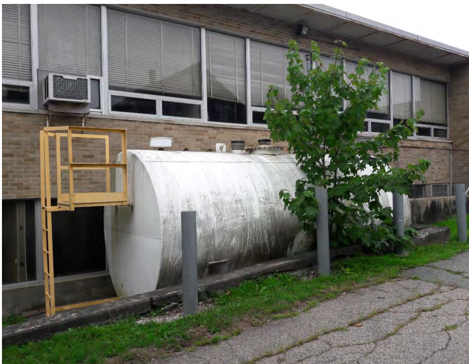
View of the heating oil AST located along the northern exterior of Building #2.
