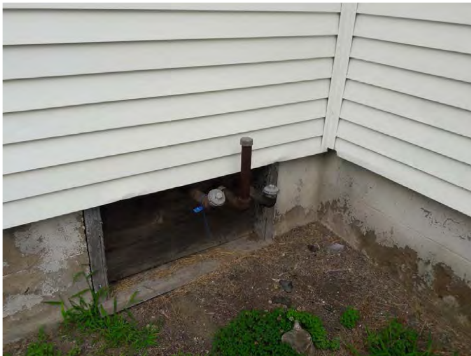
View of the fill and vent pipes associated with the aboveground storage tanks (ASTs) located in the basement of Building #1.
