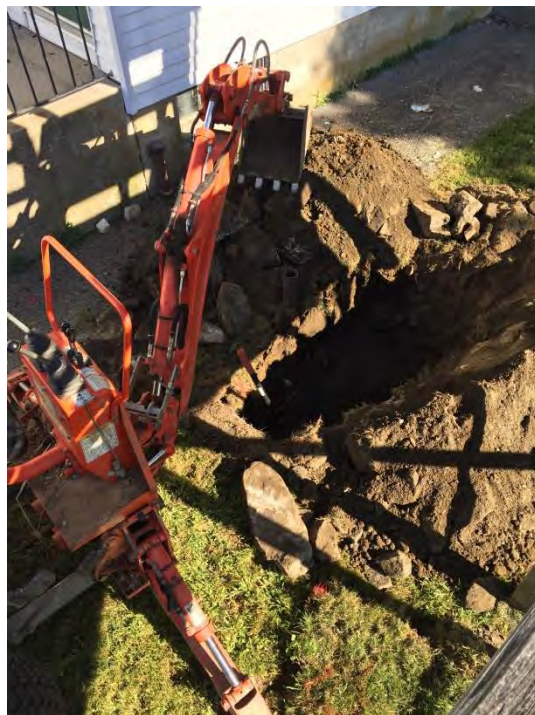
Additional view of test pit advanced within area of suspect UST near Building #1.
