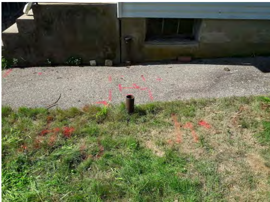
View of apparent fill and vent pipes associated with a suspected, abandoned underground storage tank (UST).
