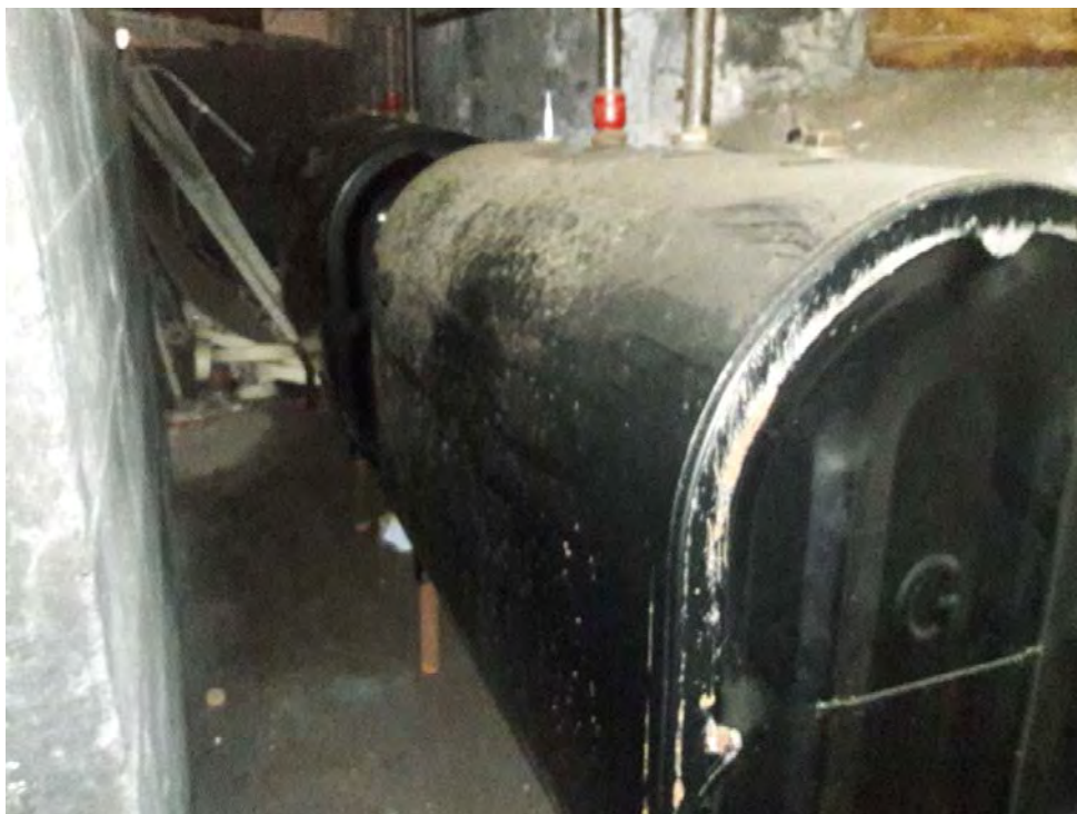
View of the two (2) active ASTs located in the basement of Building #1.
