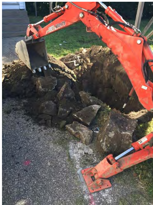
View of the test pit advanced within area of suspect UST near Building #1 (note rocks).
