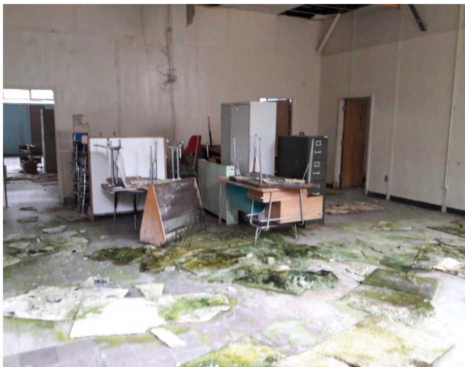
Additional view of water damage and mold located within Building #2.
