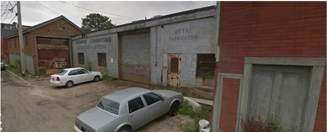
Two Views of Building at 20 West Extension Street
