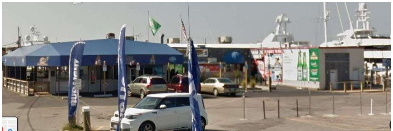
Building at 25 Waite's Wharf
