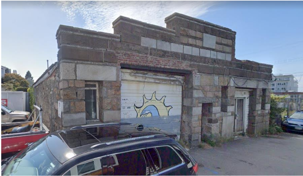
Building at 16 Waite's Wharf
