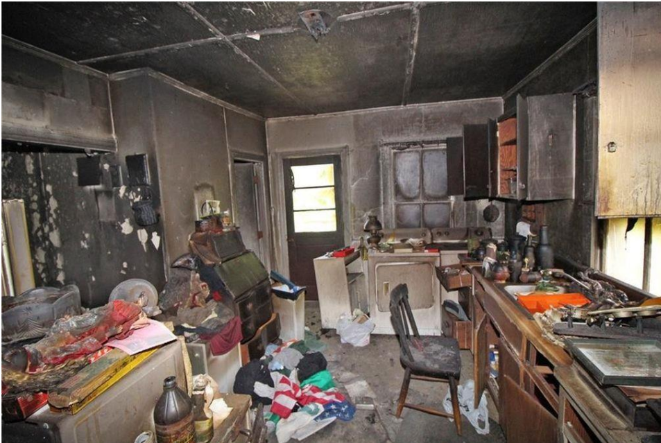
Interior smoke / fire / heat damage in first floor
