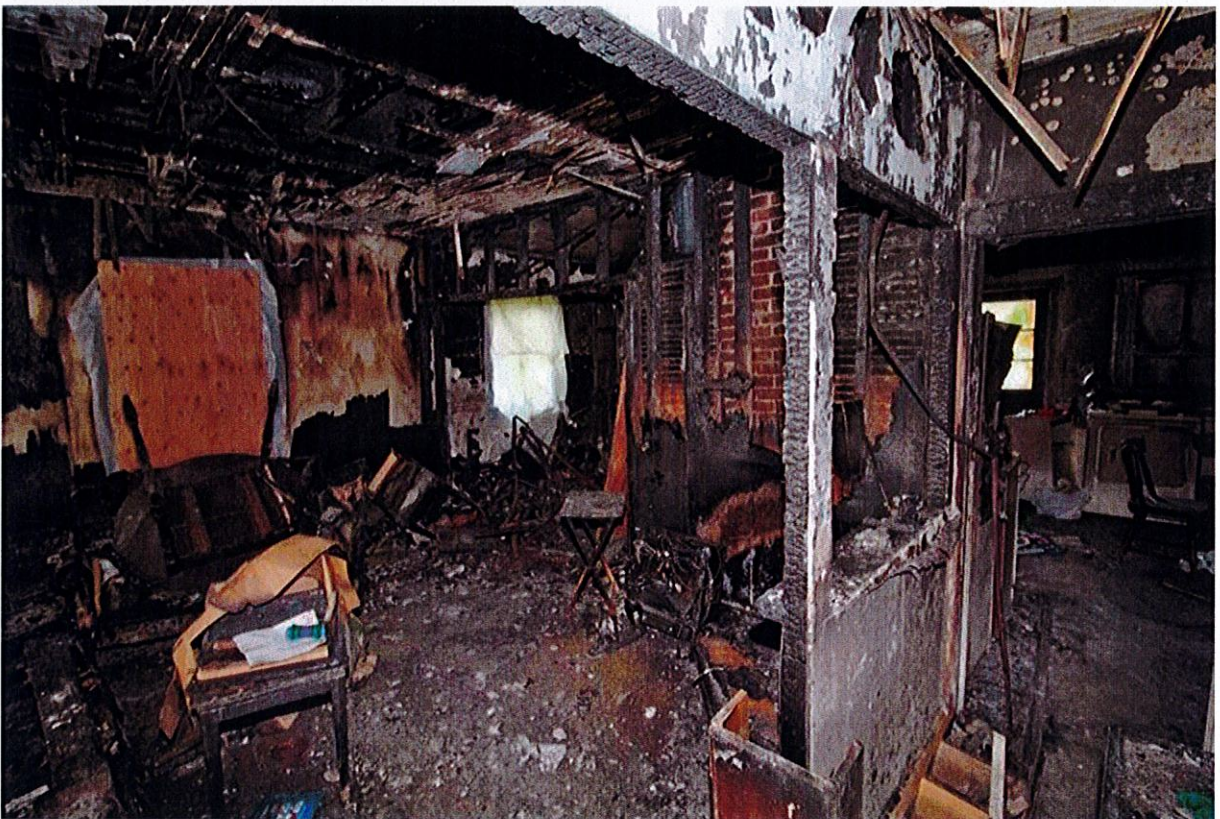
Interior smoke / fire / heat damage in first floor Note fire damaged 2 nd floor joists
