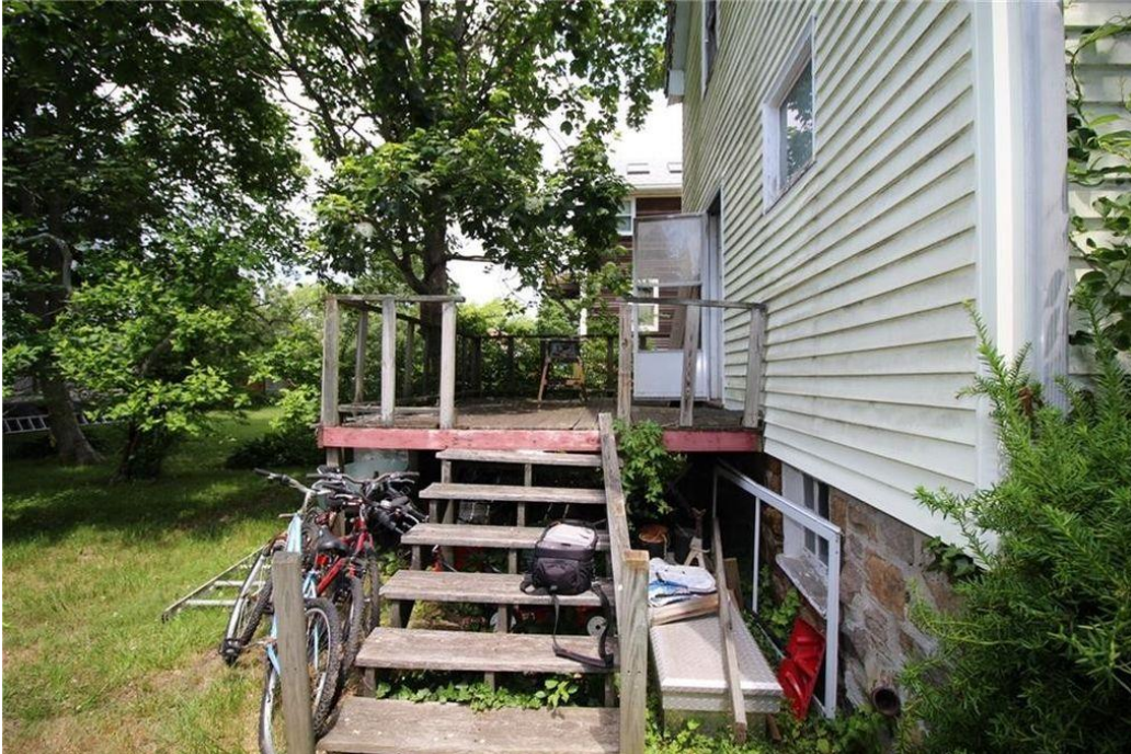
Photo of failing rear deck, railings, stairs
