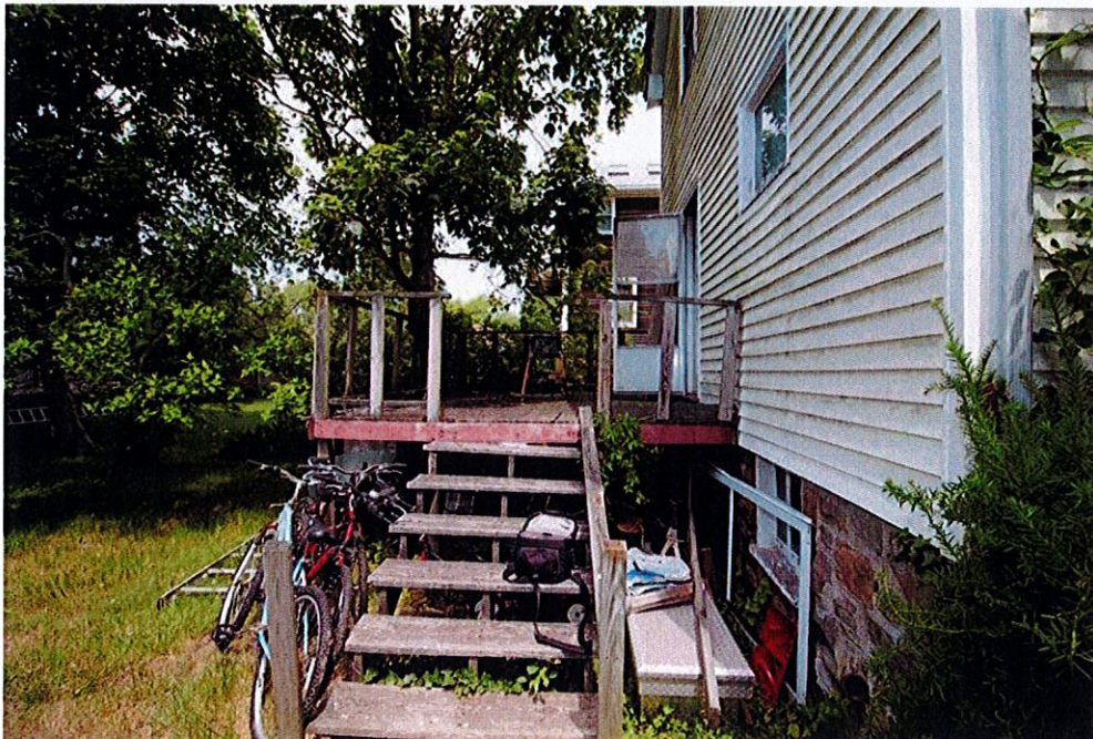
Photo of failing rear deck, railings, stairs
