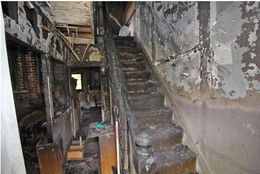
Interior smoke / fire / heat damage in first floor hallway Note tight steep main stairwell
