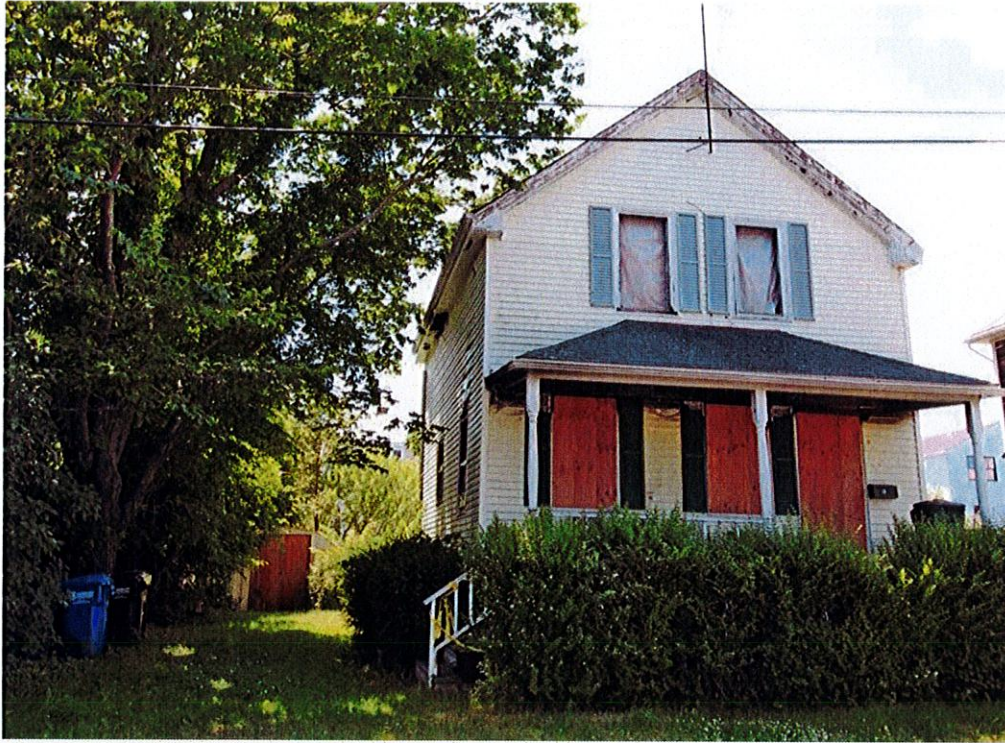
Photo of front of house (boarded up and broken windows/doors)
