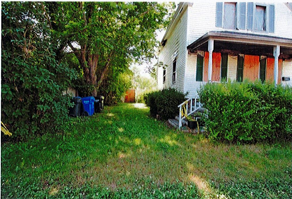
Melted siding, fire damage through upper eaves, boarded up windows/doors
