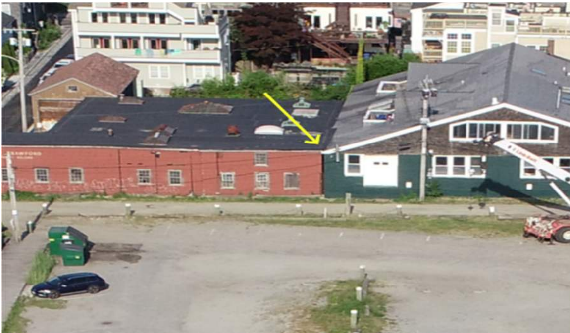
Photo 4: This photo shows the roof sheathing of sections B and C is connected to the adjacent “Casey” building. Although the sheathing is connected, this is a “non-structural” connection that can be easily severed prior to site demolition. While caution is required to demolish the Crawford The building, with respect to the Casey building, there are not physical or structural entanglements and demolition can be undertaken by a qualified contractor.
