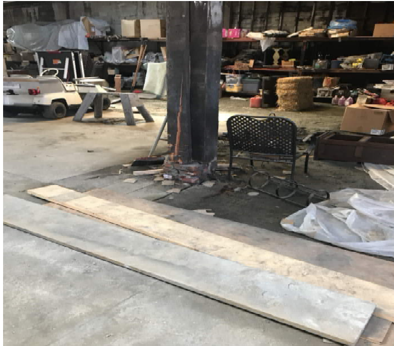
Photo 3: The photo shows the base of a wood column in section C. The wood post has a substantial crack in its base and it is also bearing on a poorly constructed brick masonry pier.
