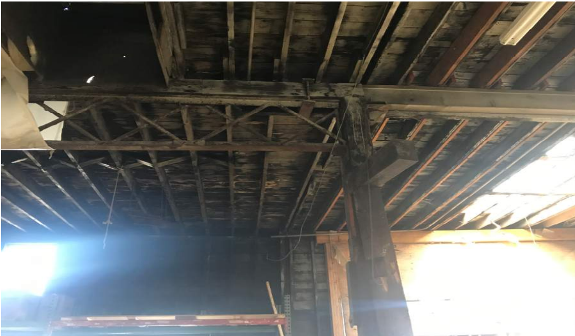
Photo 2: This photo shows a portion of the roof framing in section C. Large portions of the roof decking appear to be rotted along with a many of the roof joists. The sistered roof joists are a clear indication there was significant deterioration to the roof framing at some point. Additionally, as a
