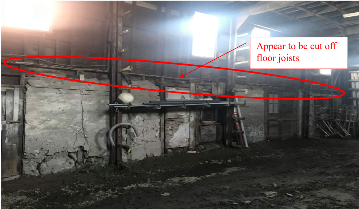
Photo 1: This photo shows the northern wall of building section A. The existing wall is comprised of multiple materials including concrete and wood. The wood framing is in direct contact with the dirt floor and this appears to be the cause for much of it to have deteriorated. The concrete portions of the wall are in significant disrepair. There are evident cracks, spalls and areas of poor consolidation. The concrete is also in direct contact with the wood framing. The existing wood framing is not rated for direct contact with concrete or soil. Finally, there appears to be evidence this building had an additional floor that was removed at some point in time. If it existed, the floor was providing bracing for the perimeter wall studs. Removal of the existing floor results in a hinge point in the wall and renders the wall deficient to resist wind loads.
