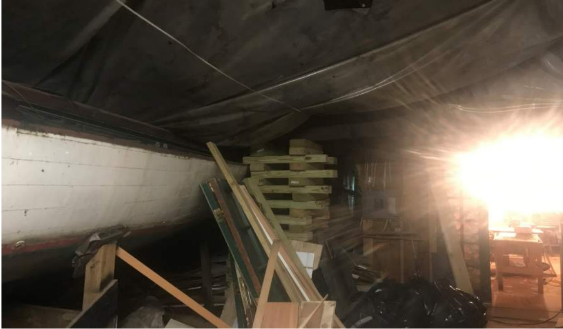
Photo 1: This photo shows cribbing supporting a collapsed roof truss in the southern portion of the building. There is also a large section in this area that has a plastic covering to help mitigate the leaking roof.
