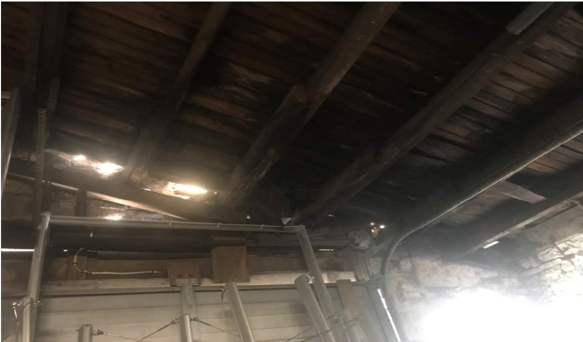
Photo 2: This photo shows northern gable end wall of the building. It is clear in this photo the building envelope is no longer in-tact and has exposed the framing to the elements. Large sections of the existing roof decking appear rotted and/or have already failed. The majority of the roof purlins also appear rotted and/or damaged. The ledger against the masonry wall has failed over the right side of the garage door opening.
