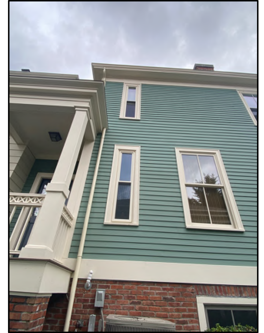
WEST ELEVATION FIRST FLOOR REMOVE EXISTING VINYL 1 OVER 1 DOUBLE HUNG WINDOW. NEW SIDING TO MATCH EXISTING
