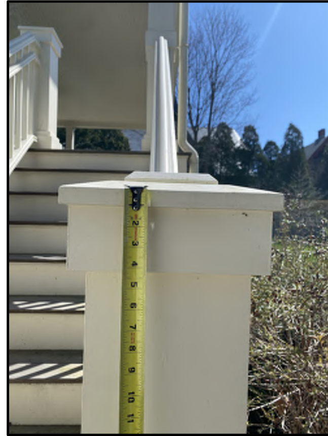
WEST ELEVATION GROUND FLOOR REAR DECK EXISTING NEWEL POST CAP TO BE MATCHED
