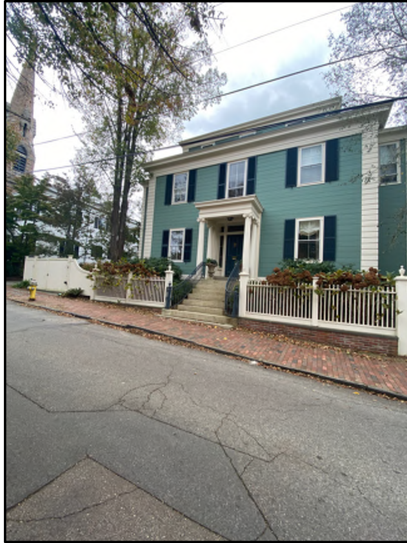
NORTH ELEVATION FRONT FACADE - NO WORK
