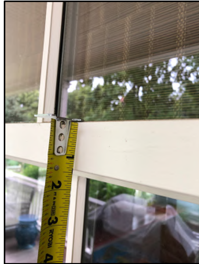
EAST ELEVATION FIRST FLOOR FAMILY ROOM EXISTING DOUBLE HUNG WINDOW LOCK RAIL/MEETING RAIL
