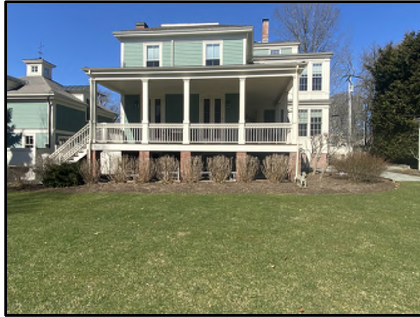
SOUTH ELEVATION GROUND FLOOR REAR DECK EXISTING DECK BALUSTRADE TO BE MATCHED
