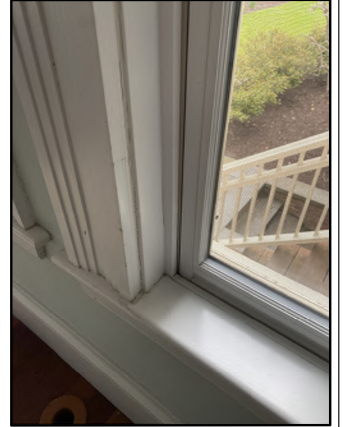
SOUTH ELEVATION FIRST FLOOR SUNROOM EXISTING DOUBLE HUNG WINDOW INTERIOR SILVER METAL SPACER BAR DETAIL
