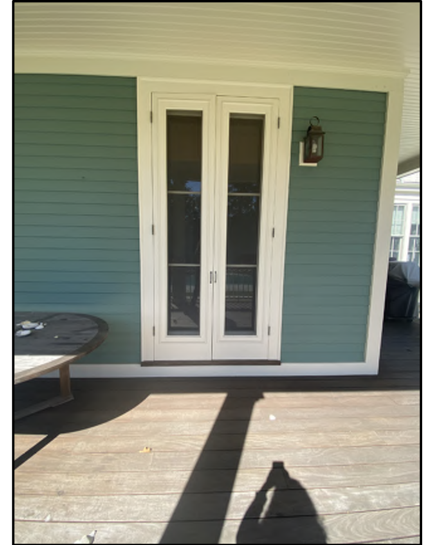
EAST ELEVATION FIRST FLOOR EXISTING FRENCH DOORS
