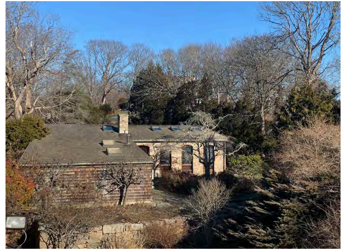
SHEEP SHED AND GARAGE, AERIAL
