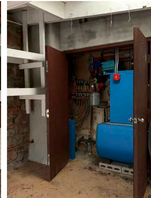
GARAGE, EXISTING EQUIPMENT
