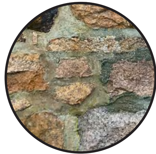
EXISTING STONE WALL, REPAIRED IN KIND
