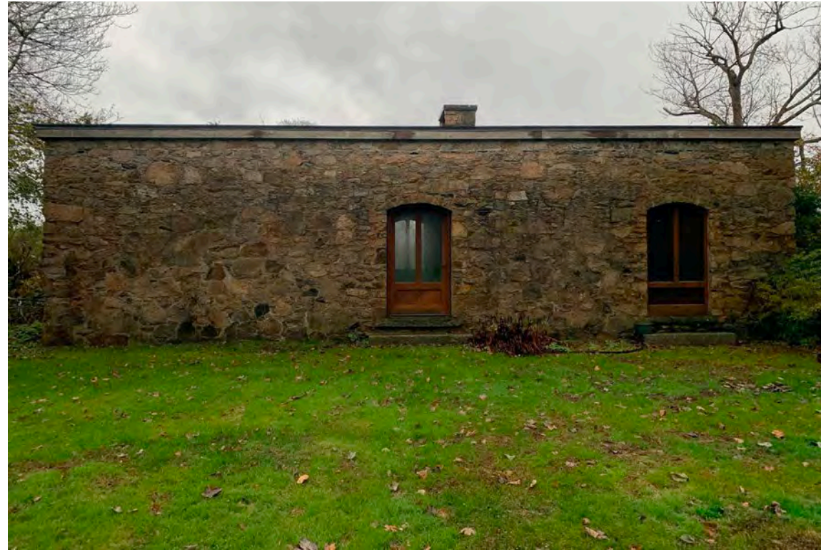
SHEEP SHED, NORTH ELEVATION
