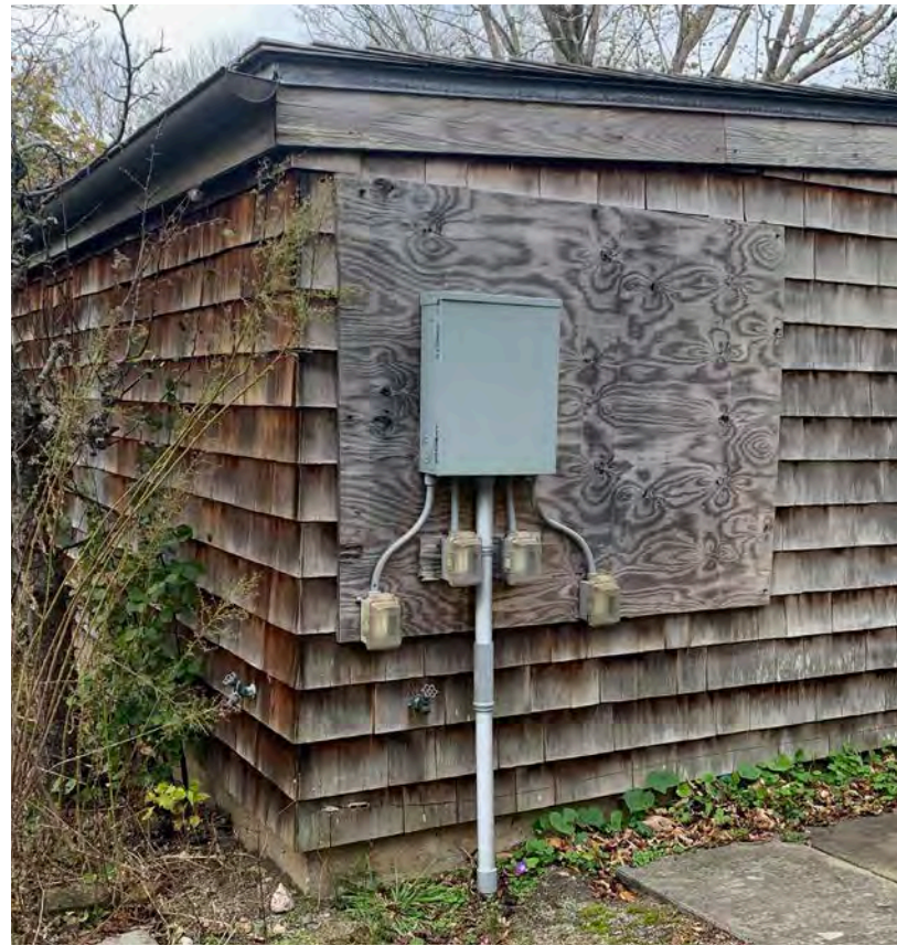
GARAGE, SE CORNER
