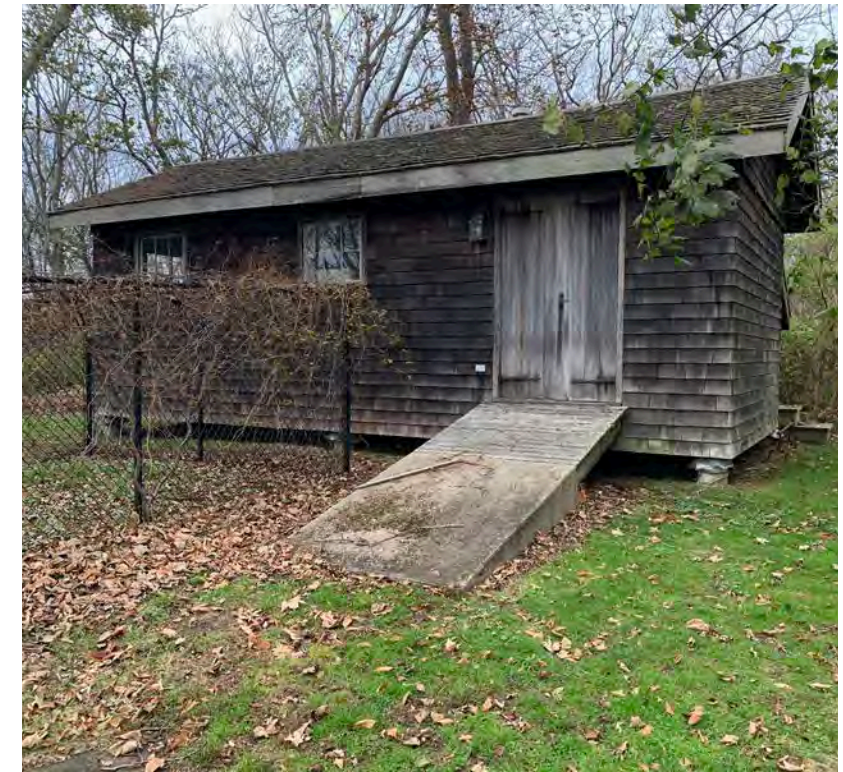
EXISTING SHED, LOCATED IN NE CORNER OF SITE
