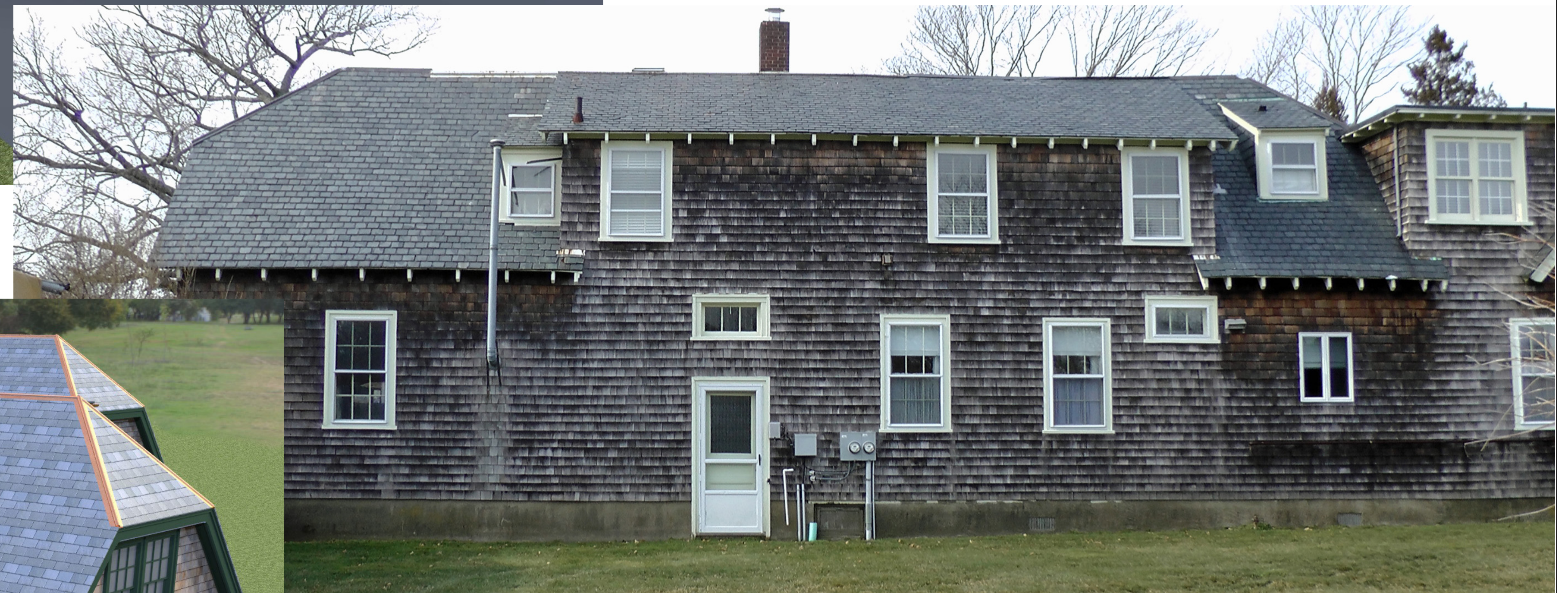
EAST PHOTO - AS-BUILT
