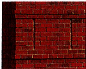
3/4" GLEN GERY BRICK VENEER CHIMNEYS
