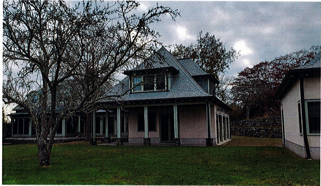
C1 VIEW AT EXISTING GARAGE FROM NORTH NOT TO SCALE
