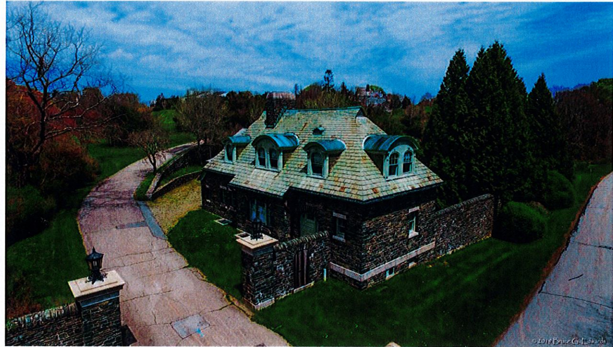
C1 EXISTING GATEHOUSE - STREET VIEW NOT TO SCALE
