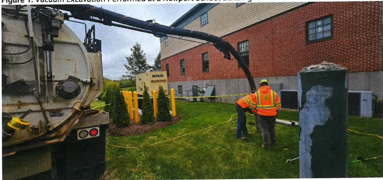
Figure 1. Vacuum Excavation Performed at a Newport School Building
