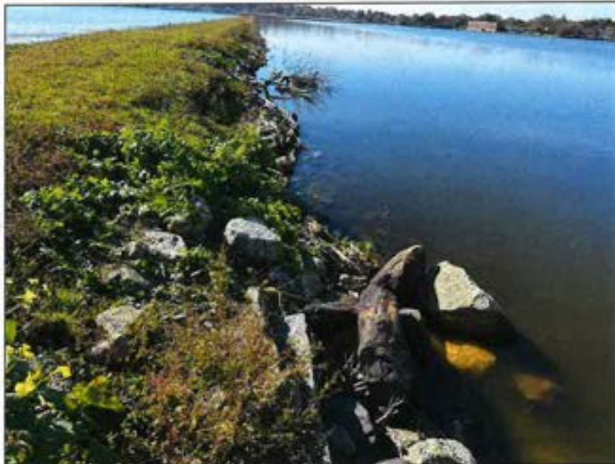
Photo No. 6.: Upstream slope from the primary spillway looking right.
