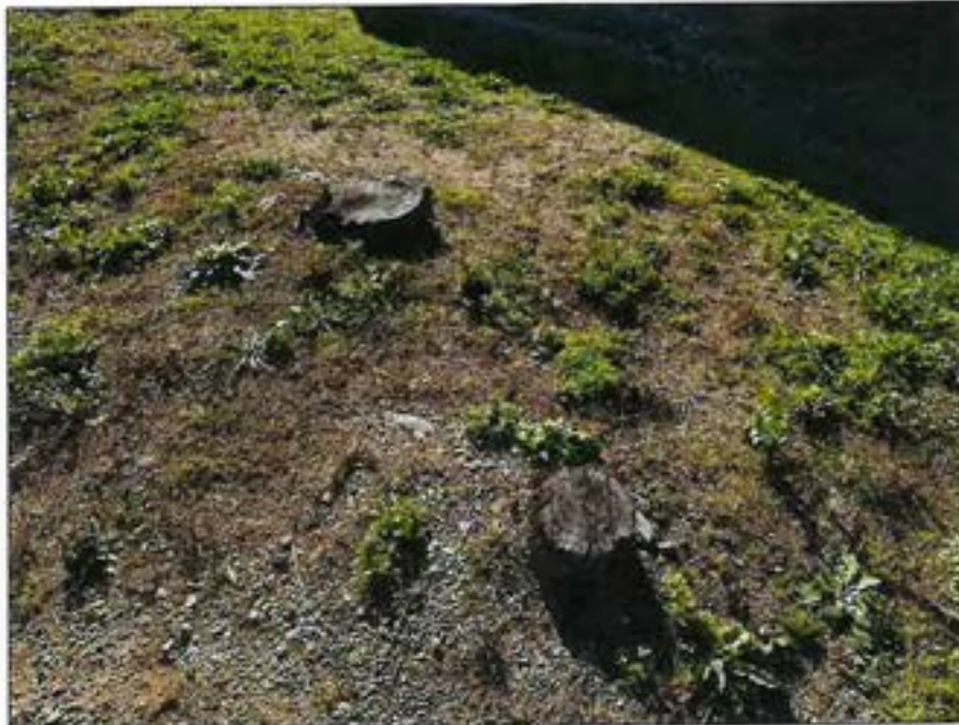
Photo No. 1.: Stumps at the right abutment.
