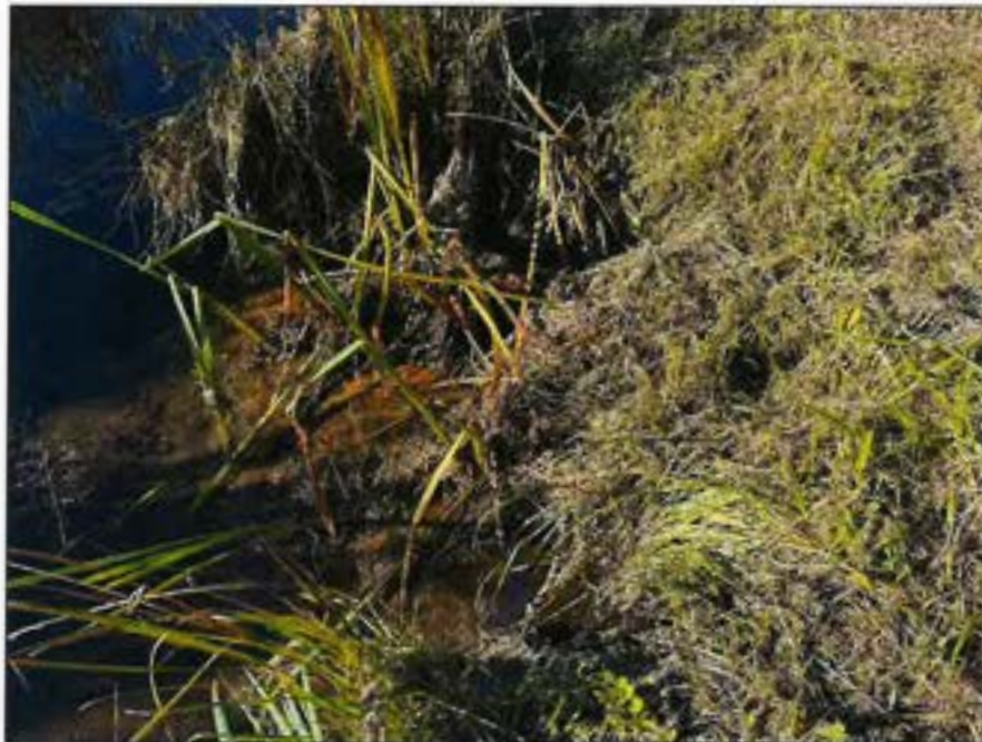
Photo No. 14.: Iron oxide stained seepage from the moat bank near STA 12+90.
