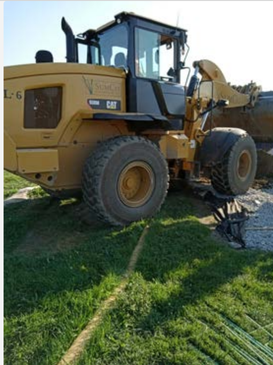
Backfill material being placed at the Right Training Wall (north end) with the CATERPILLAR 938M front-loader.
