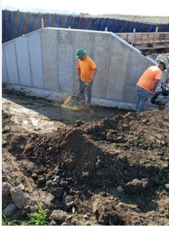
Compaction procedures underway on the Right Training Wall backfill (north end).
