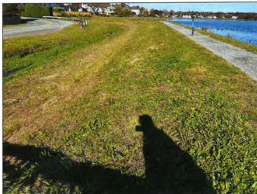
Photo No. 33.: Downstream slope from STA 37+50 looking right.
