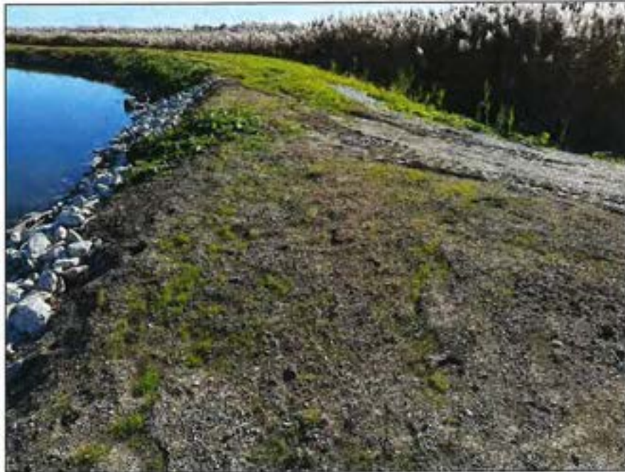
Photo No. 9.: Crest from the auxiliary spillway looking left. Note bare soils due to replacement of the auxiliary spillway.
