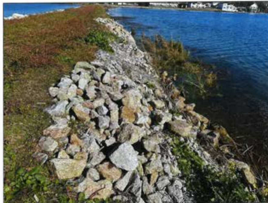
Photo No. 18.: Downstream slope near STA 18+50 looking left. Note riprap repair, typical throughout the slope.
