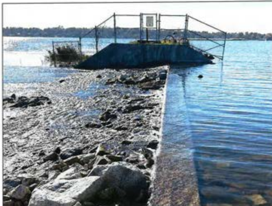
Photo No. 22.: Right training wall of the spillway. Note new surface concrete.
