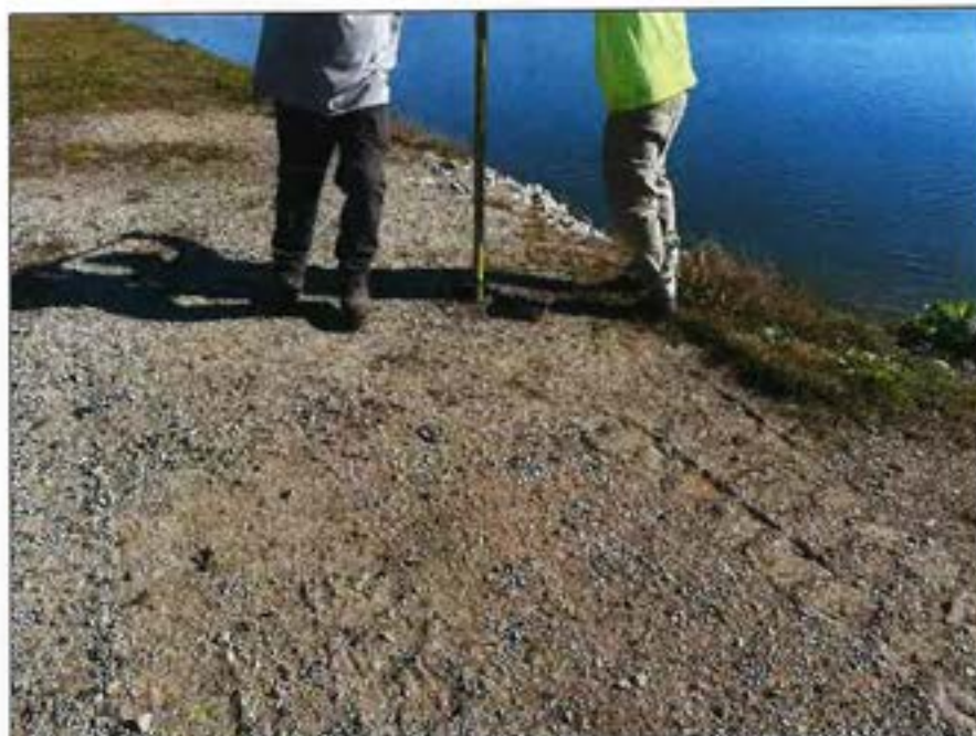
Photo No. 34.: City of Newport operating the low level outlet. Outlet is operable.
