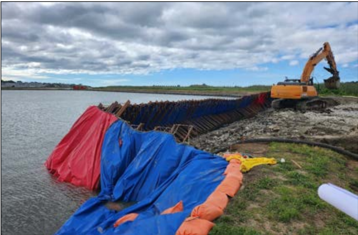
Photo 2: Overview of the Installed Portadam
