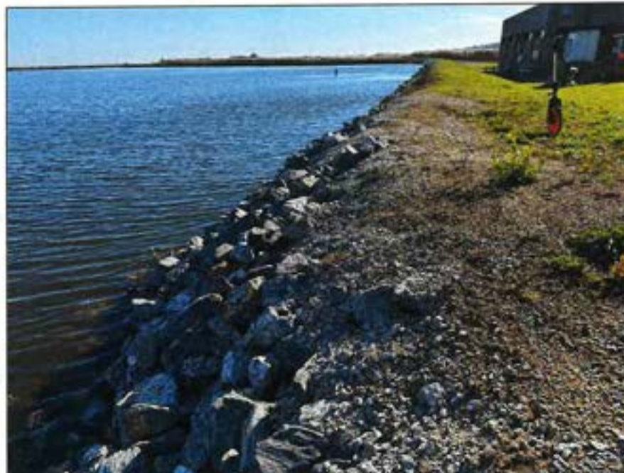
Photo No. 2.: Upstream slope from the right abutment looking left.
