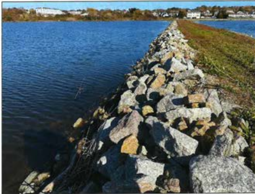
Photo No. 5.: Upstream slope near STA 18+00 looking left. Note new riprap placed along the slope.
