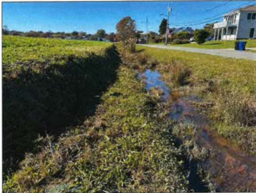
Photo No. 45.: Downstream slope from STA 70+00 looking left.
