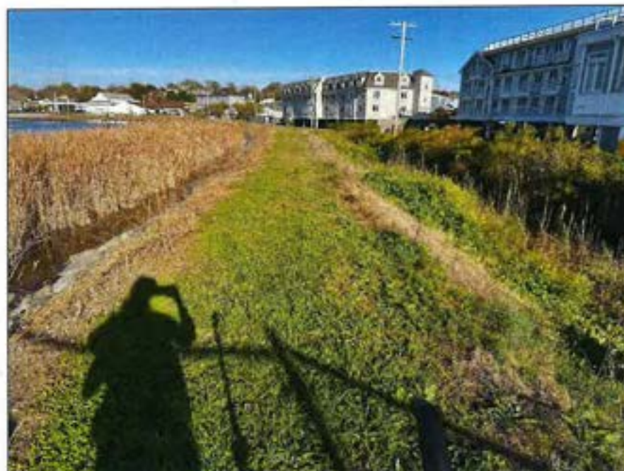
Photo No. 50.: Crest from the primary spillway looking left.
