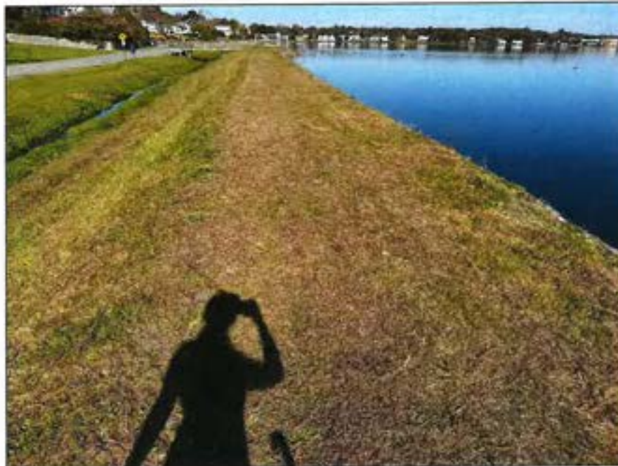
Photo No. 29.: Overview looking left near STA 32+00.
