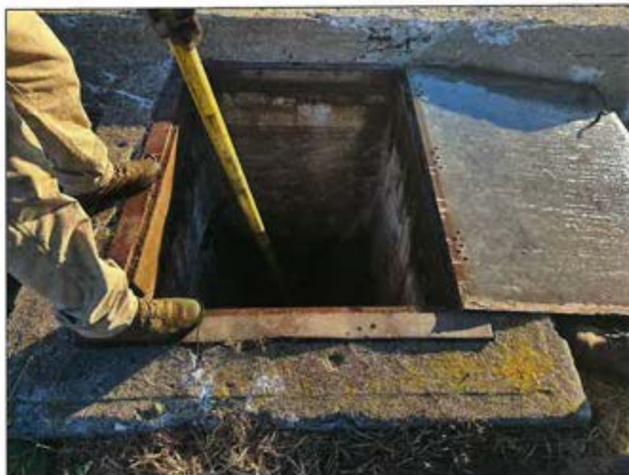
Photo No. 1.: Interior of the low level outlet chamber. Note the city operating the valve during the inspection.
