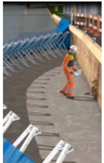
Work area dewatered
