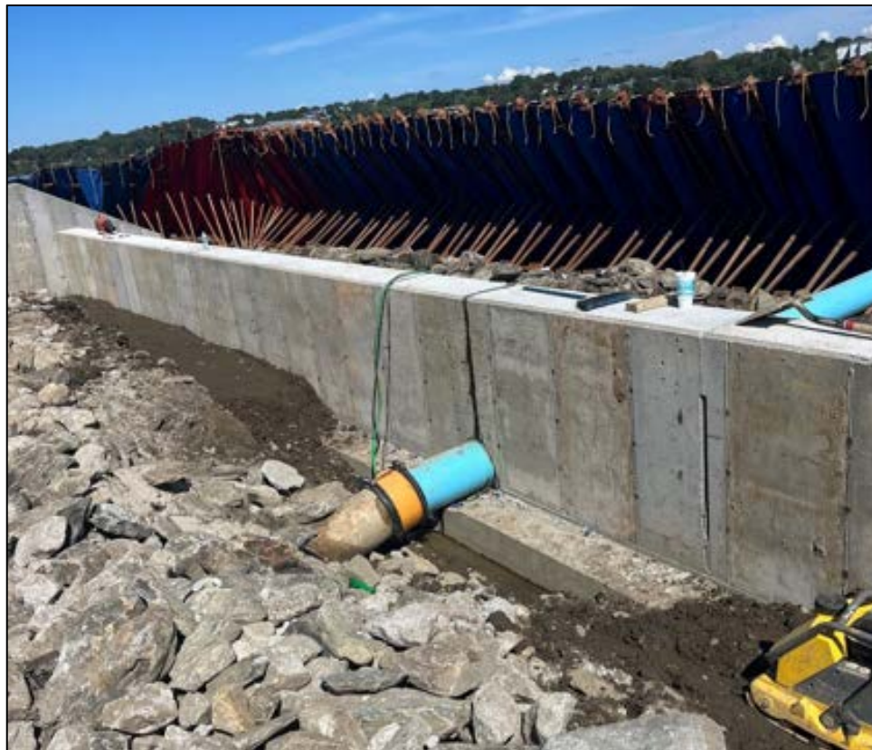
Photo 4: Overview of Wier Wall and Blowoff Pipe
