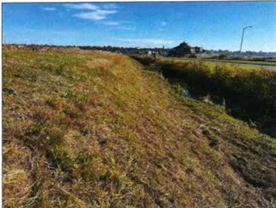
Photo No. 17.: Downstream slope from STA 18+00 looking left.
