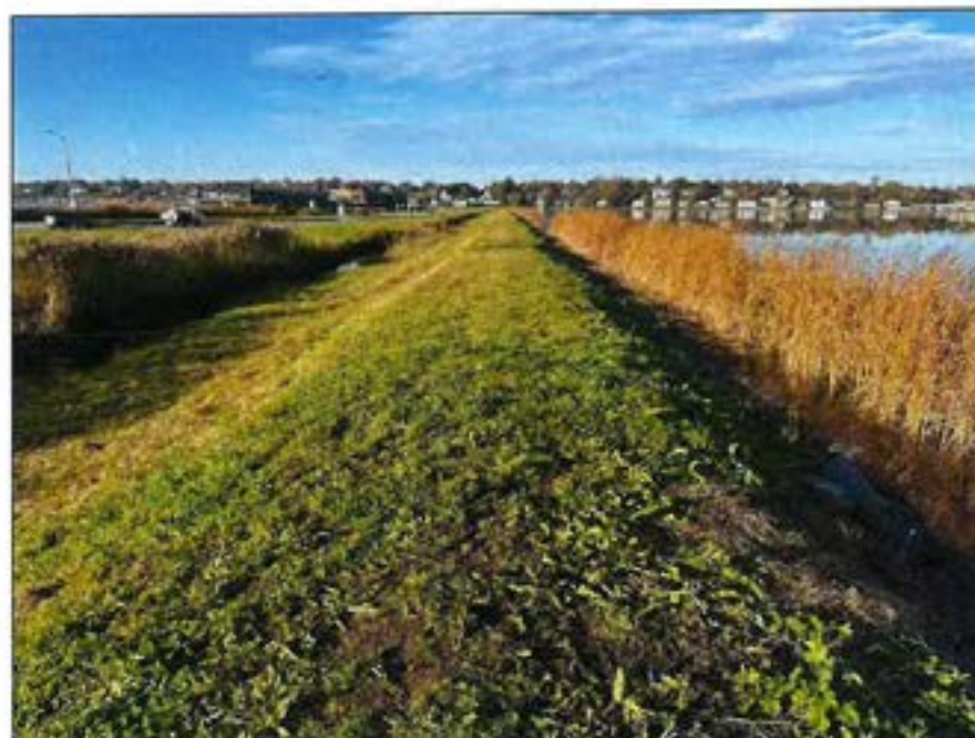
Photo No. 10.: Crest from the primary spillway looking right.
