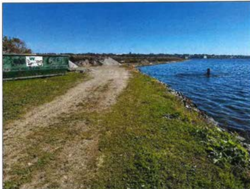
Photo No. 46.: Overview from STA 71+00 looking right.
