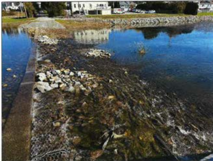
Photo No. 25.: Discharge apron of the spillway.
