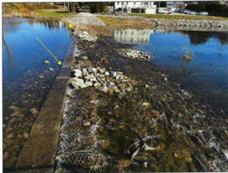
Photo No. 21.: Primary spillway from the right end looking left. Note difference in elevation of the spillway crest.
