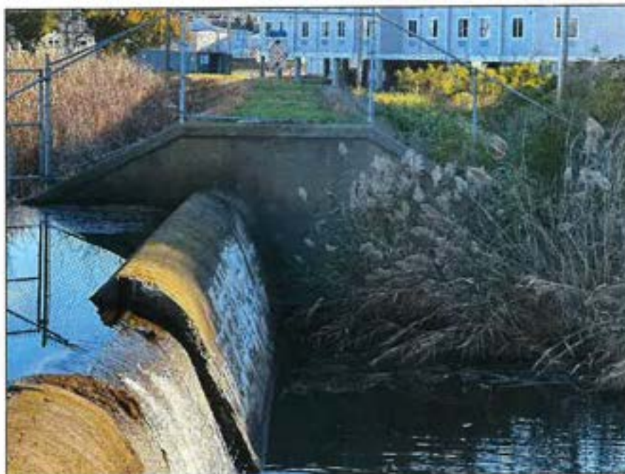
Photo No. 5.: Left training wall of the primary spillway.
