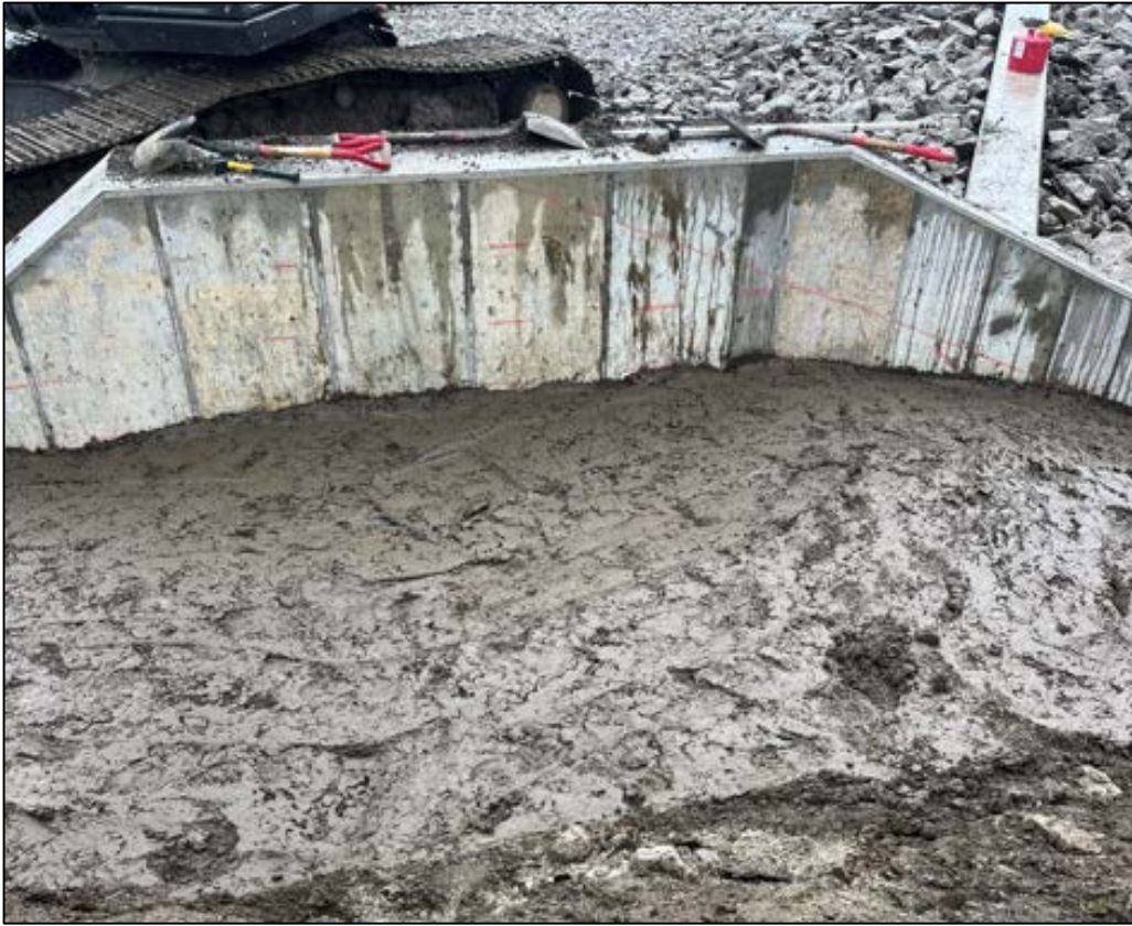
Photo 5: Backfilling Left Training Wall
