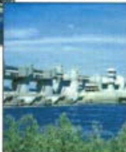
Lock and Dam
