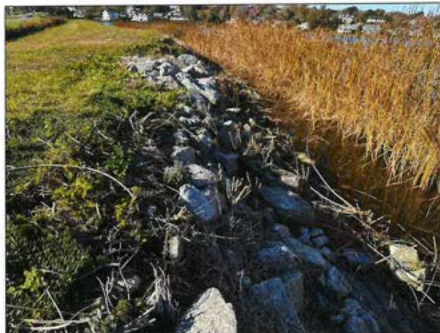
Photo No. 22.: Upstream slope from STA 18+00 looking right. Note riprap repair.
