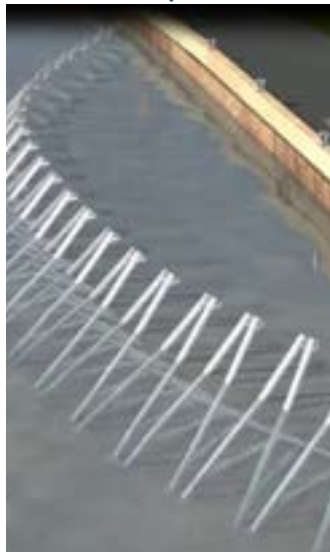
Frames set in place
