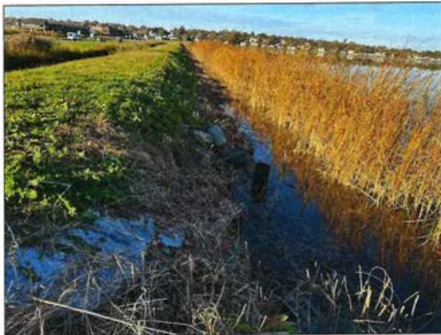
Photo No. 9.: Upstream slope from the primary spillway looking right.
