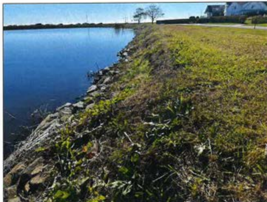
Photo No. 30.: Upstream slope looking left near STA 32+00.
