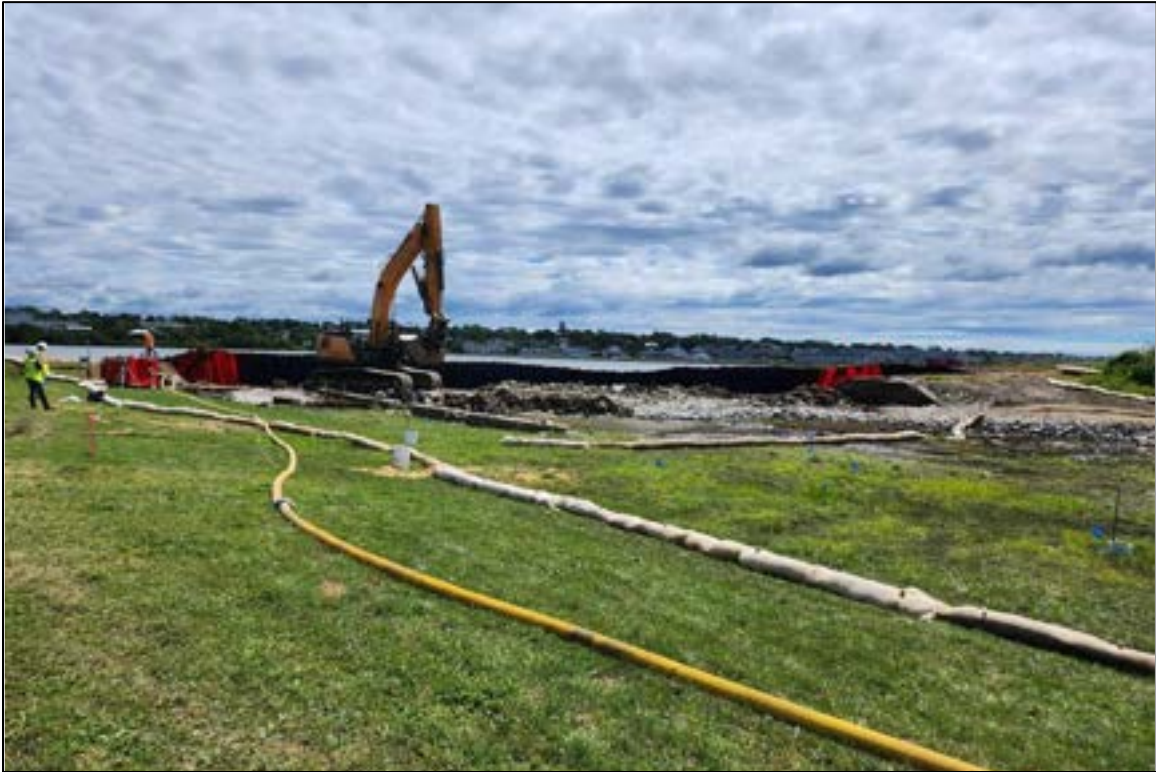
Photo 1: Overview of the Spillway at the Start of Construction
