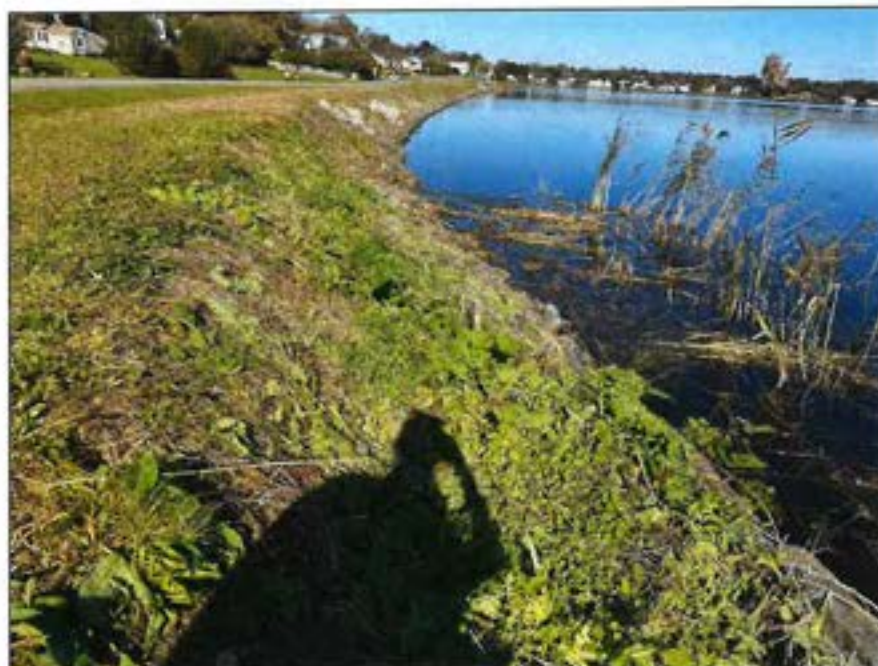
Photo No. 26.: Upstream slope from STA 30+00 looking right.
