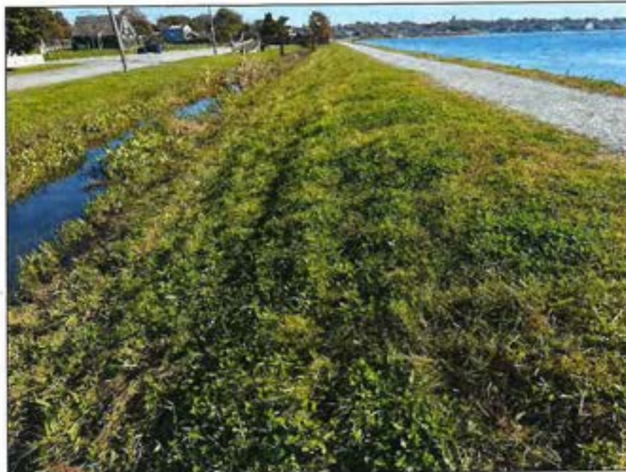
Photo No. 41.: Downstream slope from STA 58+00 looking right.
