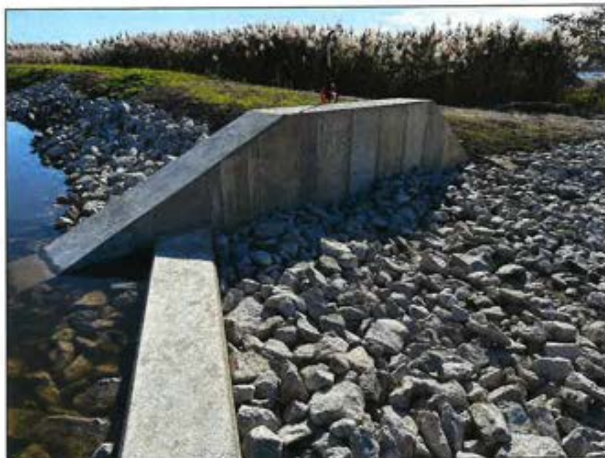
Photo No. 29.: Left training wall of the auxiliary spillway.
