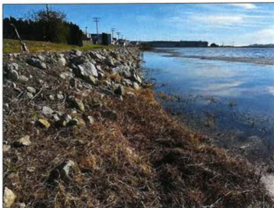
Photo No. 54.: Upstream slope of the embankment to the left of the spillway. Note repaired riprap.
