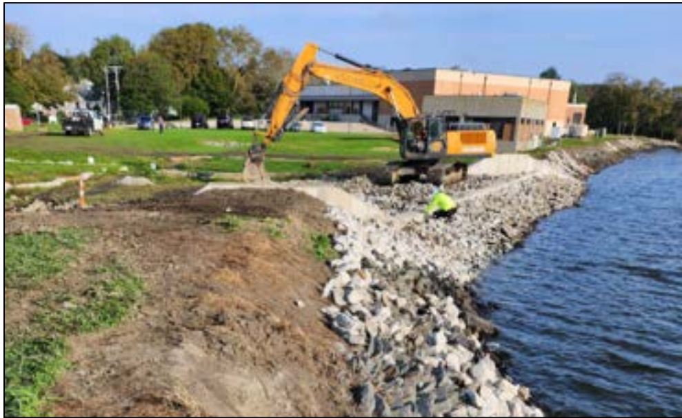
Photo 7: Overview of Auxiliary Spillway towards the End of Construction
