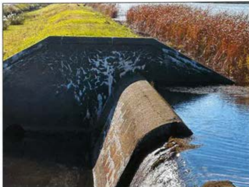
Photo No. 6.: Right training wall of the primary spillway.
