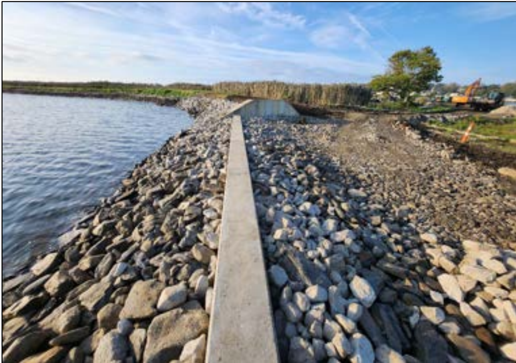
Photo 6: Overview of Left Training Wall and Weir Wall towards the End of Construction
