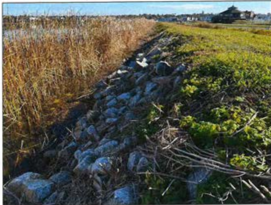
Photo No. 21.: Upstream slope from STA 18+00 looking left.
