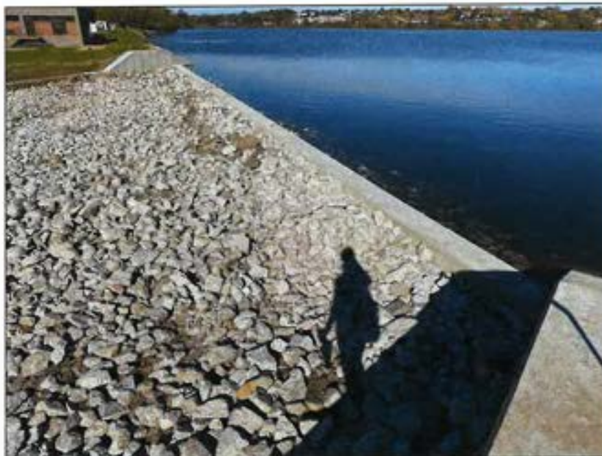
Photo No. 26.: Auxiliary spillway from the left end looking right.
