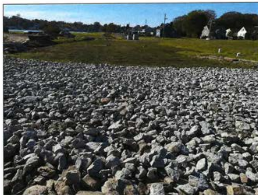
Photo No. 30.: Discharge of the auxiliary spillway.
