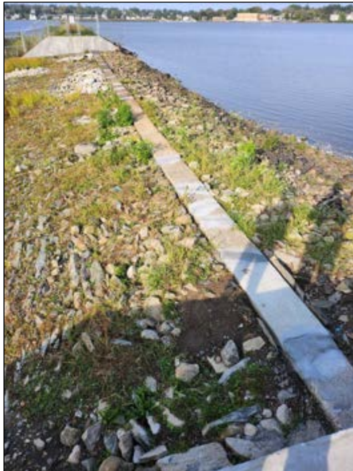
Photo 8: Overview of Repairs to the Primary Spillway
