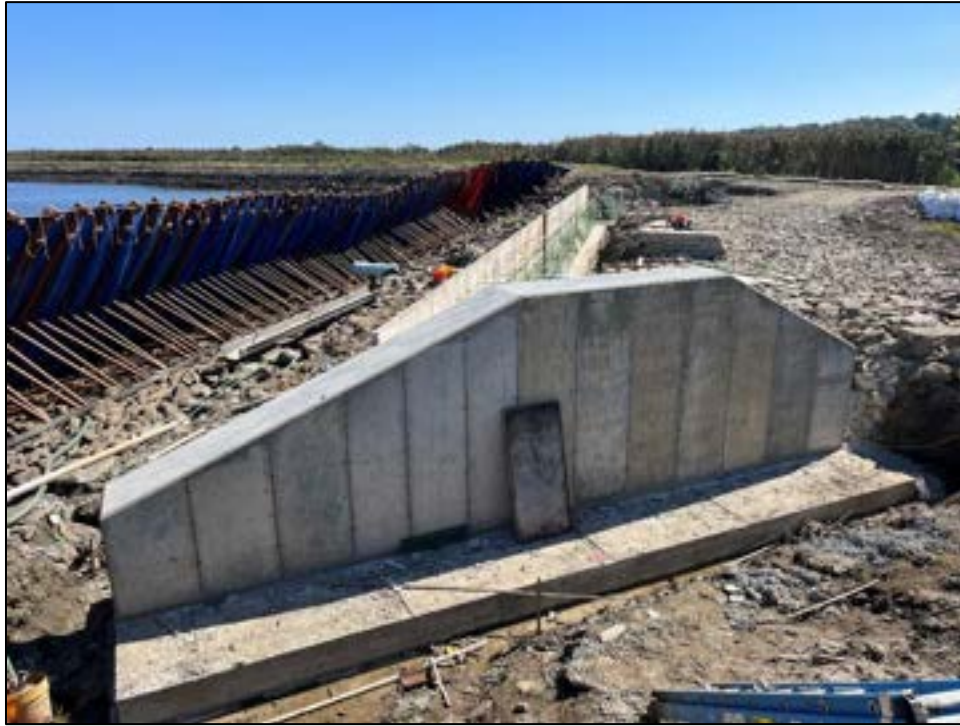
Photo 3: Overview of Right Training Wall
