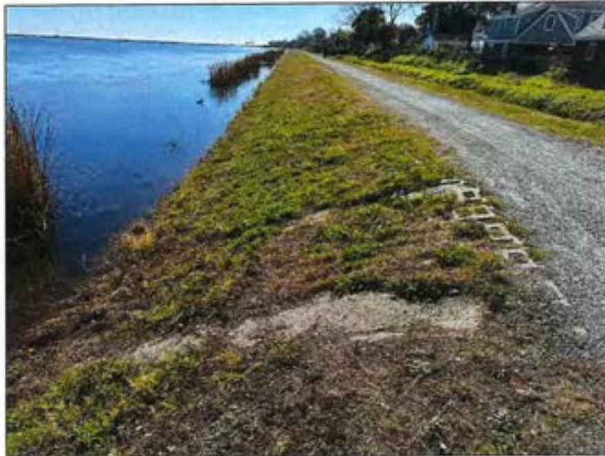
Photo No. 37.: Upstream slope from STA 57+00 looking left.
