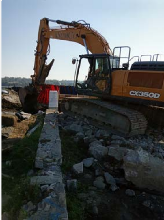
Backfill material being leveled with the CX 350D excavator bucket.
