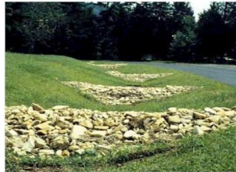
Typical Bioswale Source: Pennsylvania Stormwater Manual Section 6.4.8
