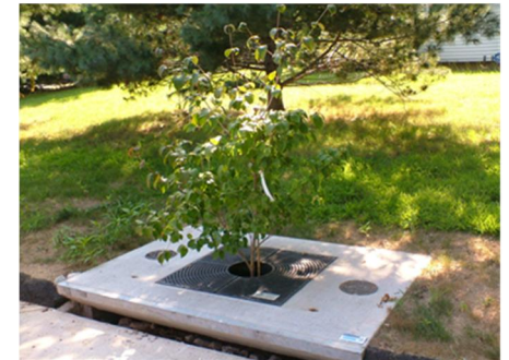
Example Tree Filter Source: CTDEEP, http://www.ct.gov/deep/cwp/view.asp?A=2719&Q=567354
