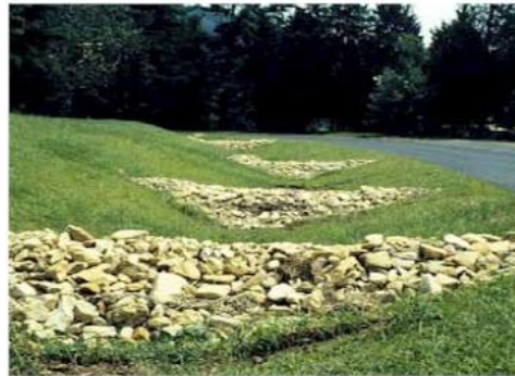
Typical Bioswale Source: Pennsylvania Stormwater Manual Section 6.4.8
