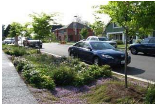
Typical Roadside Bioswale Source: USEPA, https://www.epa.gov/green-infrastructure/what-green-infrastructure
