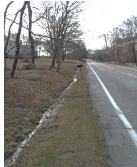
Existing Swale - East Main Road Source: Fuss & O'Neill, 2016
