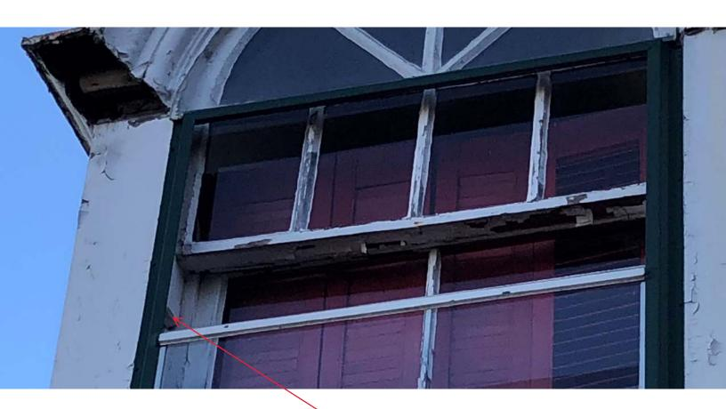
Block in window jamb holding upper sash closed
